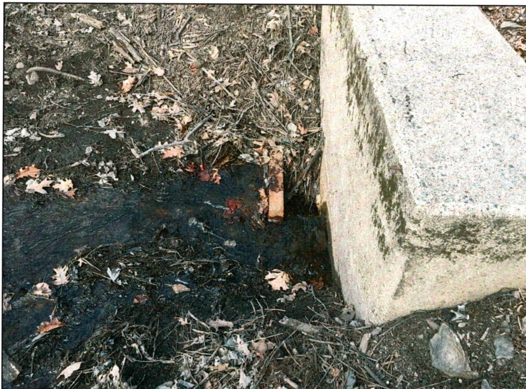
Photo No. 4: View of headwall and pipe inlet that drains the wetland and intermittent stream. This inlet clogged and flooded the wetland on January 26 th Pare recommends regularly maintaining this inlet and installing a debris rack to prevent regular clogging.
