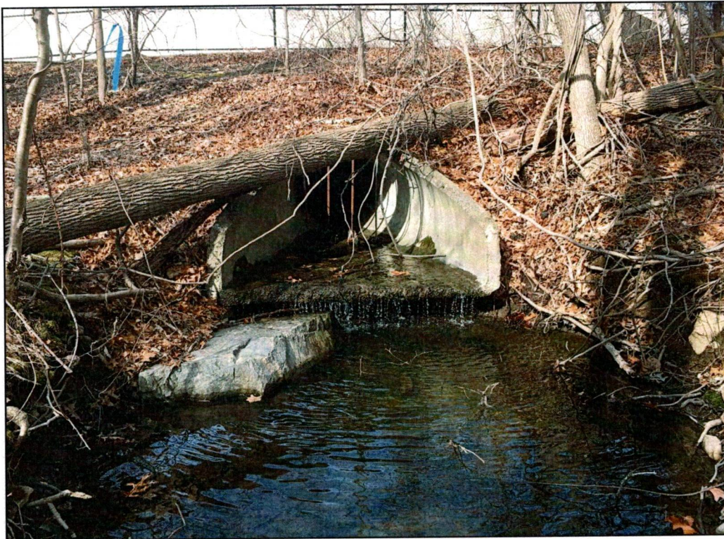
Photo No. 1: View of the 36-inch stormwater outfall from which the sediment was discharged to the wetland.
