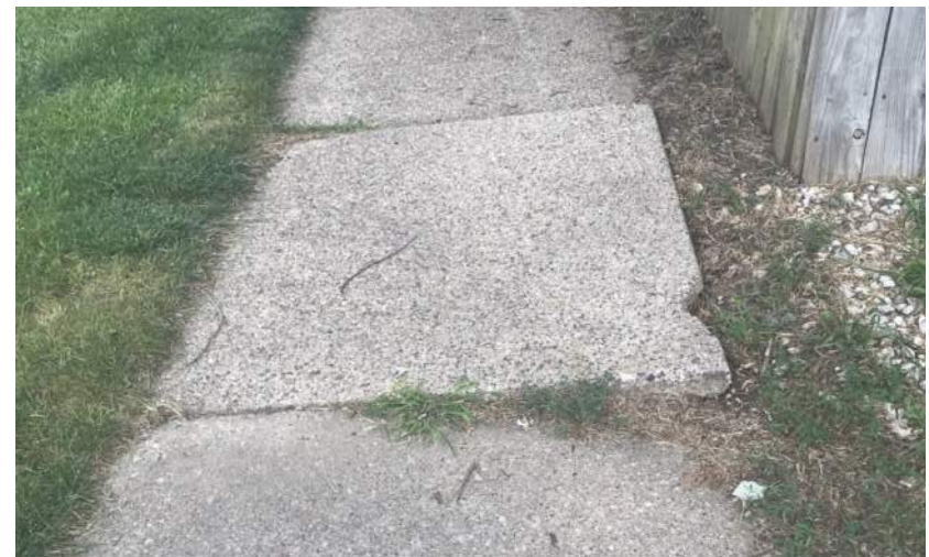
Figure 4.5: Heaved Sidewalk Panel
