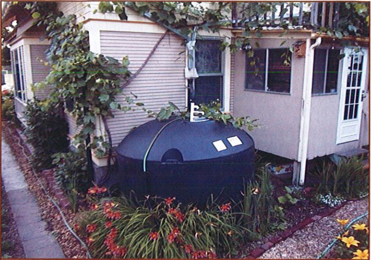
A 1500 gallon cistern fed from two gable downspouts. (Source: Experiments in Sustainable Urban Living)
