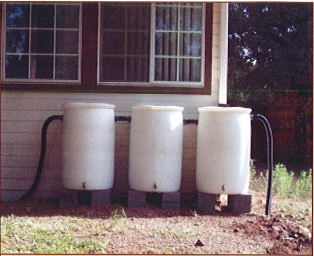
A triple set of rain barrels, connected to each other and draining to a garden or lawn area. Source: www.ne-design.net
