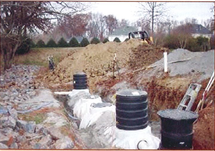
A below ground cistern installed for water harvesting storage and use. Source: Georgia Rainwater Harvesting Guidelines
