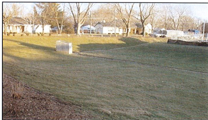
Above: Traditional storm water basin for flood control.
