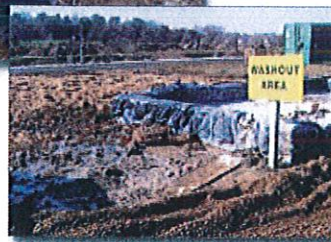
Figure 10. Leaking washout pit that has not been well maintained
