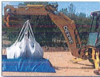
Figure 12. Extracting the concrete solids or gelled washwater
