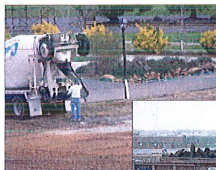
Figure 1. Chute washwater being dumped on the ground
