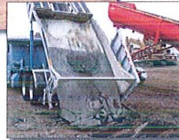
Figure 15. Delivering hardened Concrete to a recycler
