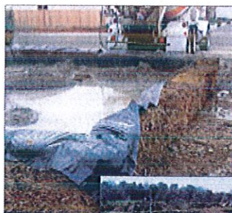
Figure 9. Hay bale and plastic washout pit
