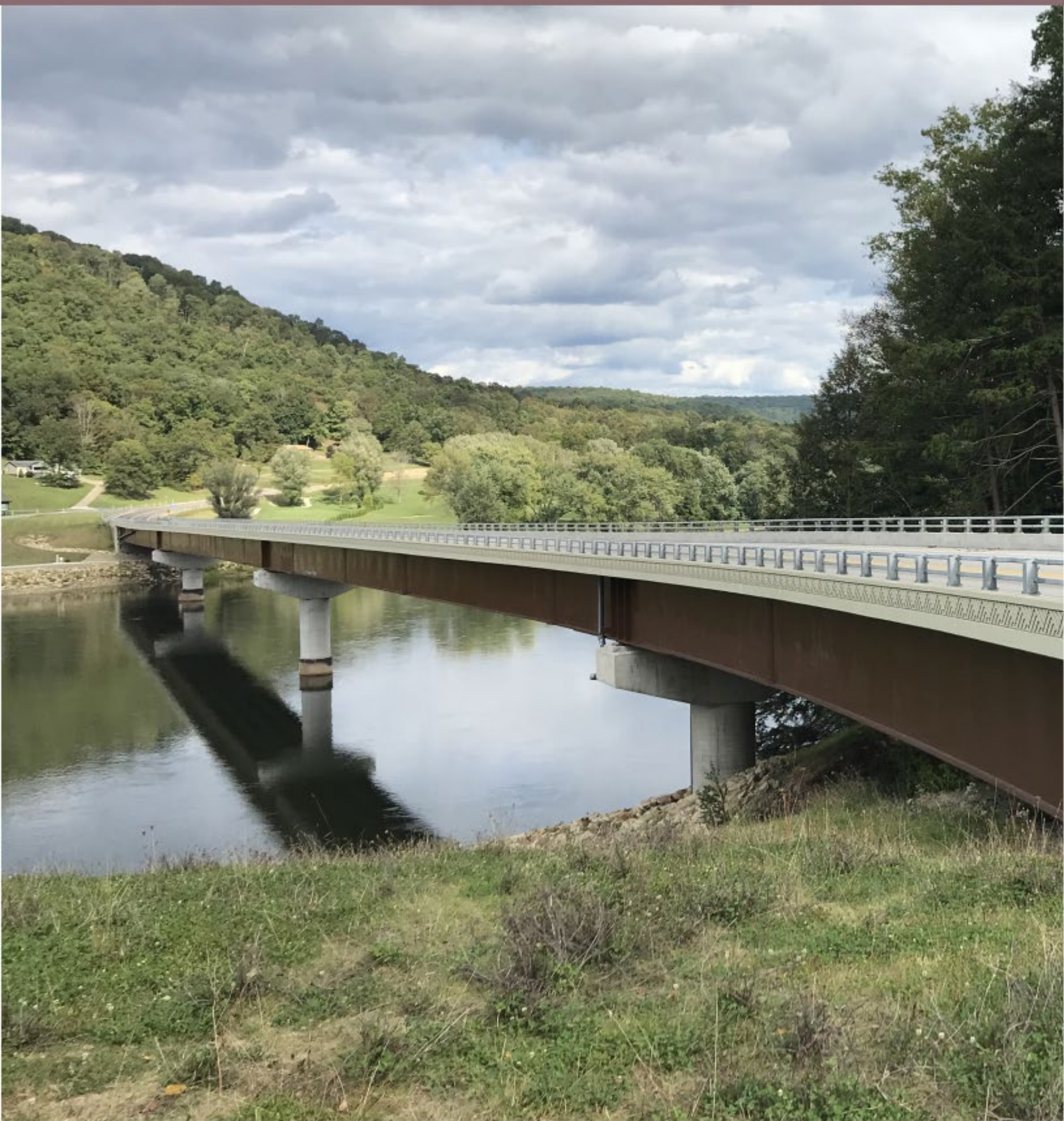
Hunter Station Bridge, carrying US 62 over the Allegheny River in Forest County
