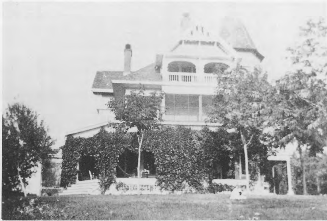
Harvard Place, home of first Newport mayor Henry James. This house was destroyed by fire.
