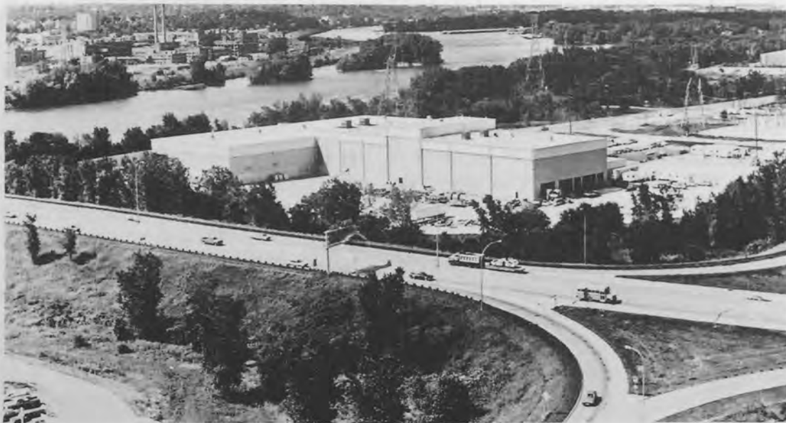
The Ramsey-Washington Refuse Derived fuel plant processes garbage into fuel
