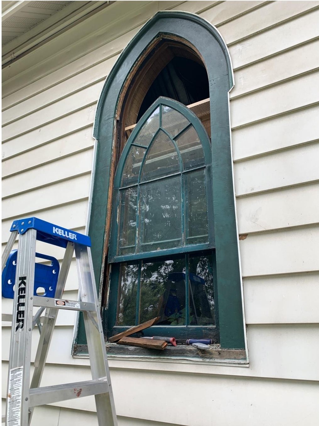
The upper sashes are still functional but have been blocked in place for many decades. Would require an operational tune-up. Notice how the sill is flush with the siding.
