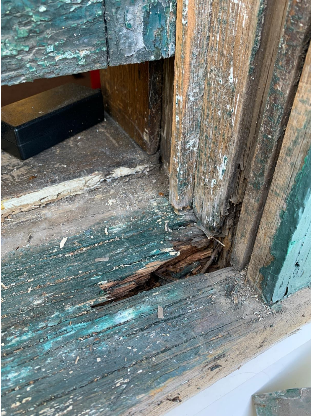
Damaged sill that requires replacement.
