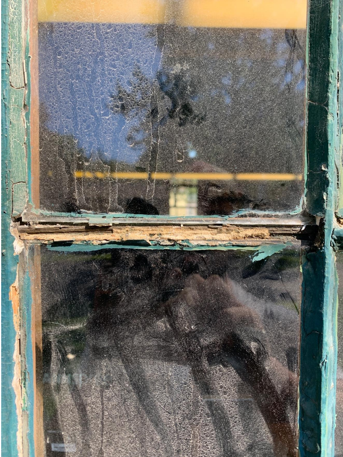
Damaged window sticking that requires replacement
