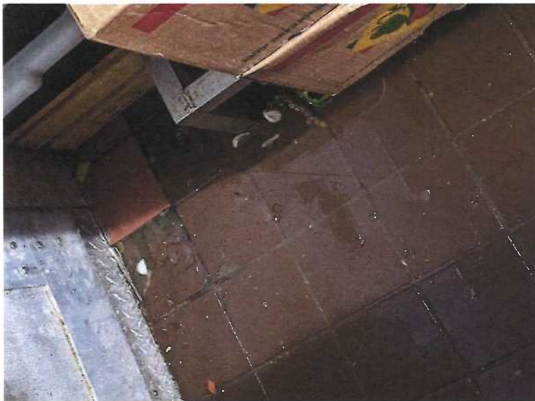
walk-in cooler floor is unclean, wet; broken floor tile
