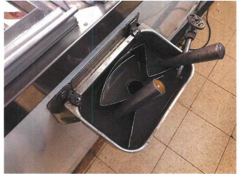
dipper well inlet submerged, causing backsiphonage risk
