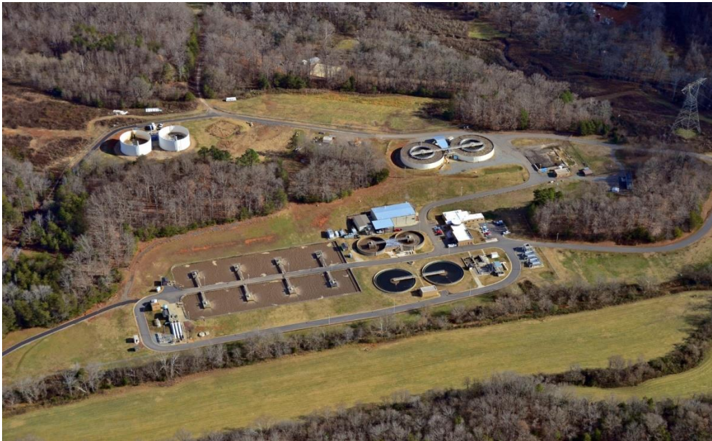
Rocky River Wastewater Treatment Plant
