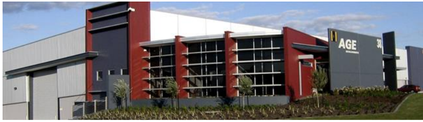
Figure 5-33: Articulation of Building Façades
