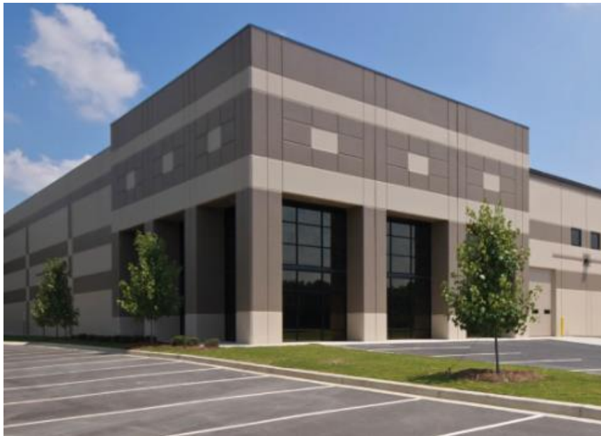
Figure 5-32: Industrial Building Entrance Features
