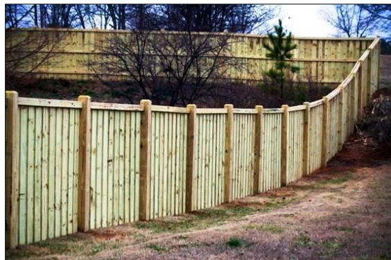
Figure 5-16: Fence with Finished Side Out
