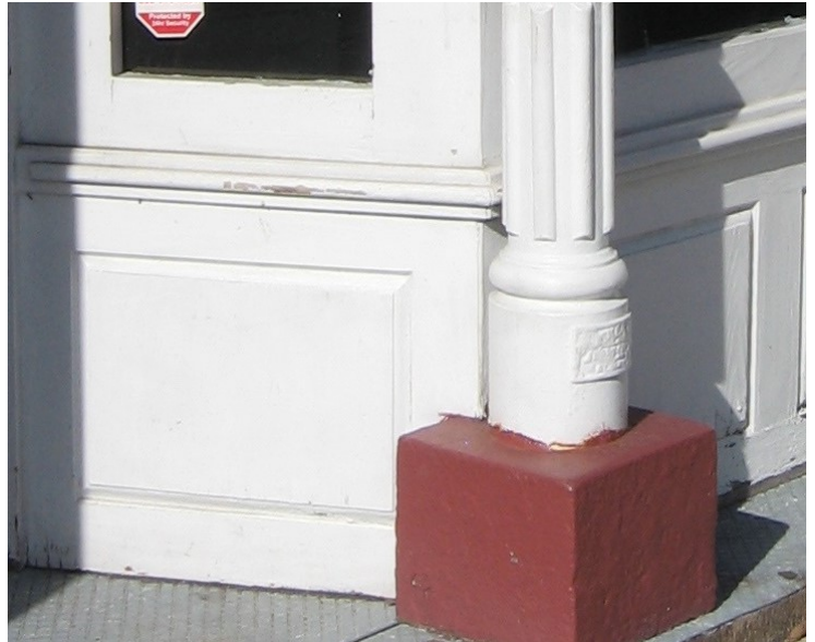
If original frame bulkheads are missing, replace them with new wood bulkheads—this replacement wood paneled bulkhead is an appropriate design.
