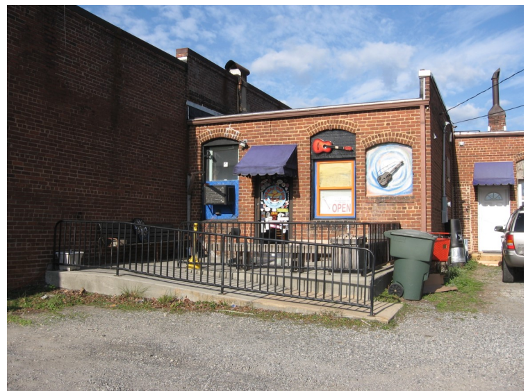
Appropriate ADA ramp located on the rear façade of this building.
