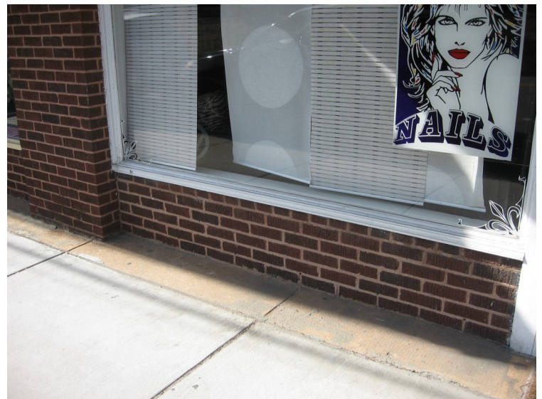
Another original brick bulkhead is on this storefront.
