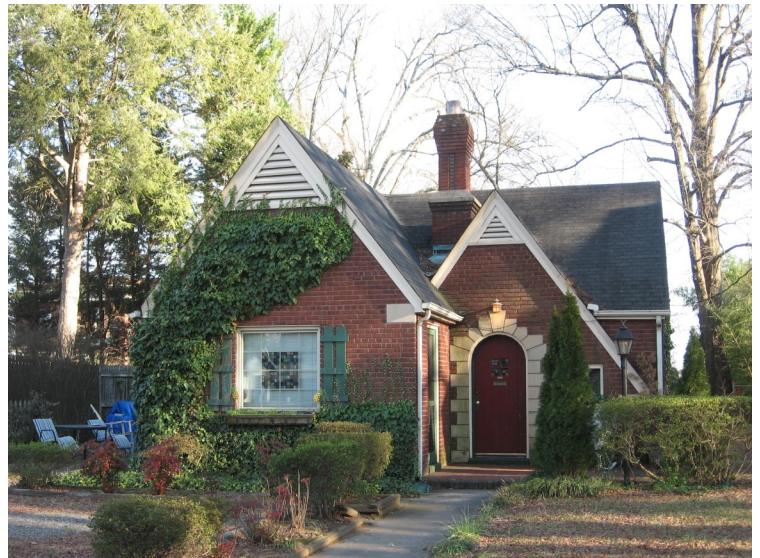
This Tudor Revival style dwelling features an arched entrance with a stone surround.
