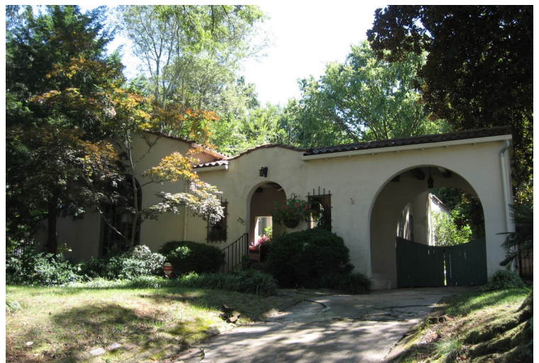
The Spanish Revival style features clay tile roofs, stucco exteriors arched entrances and open porches.
