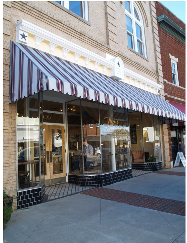
This storefront retains its angled display windows and black tile bulkheads.
