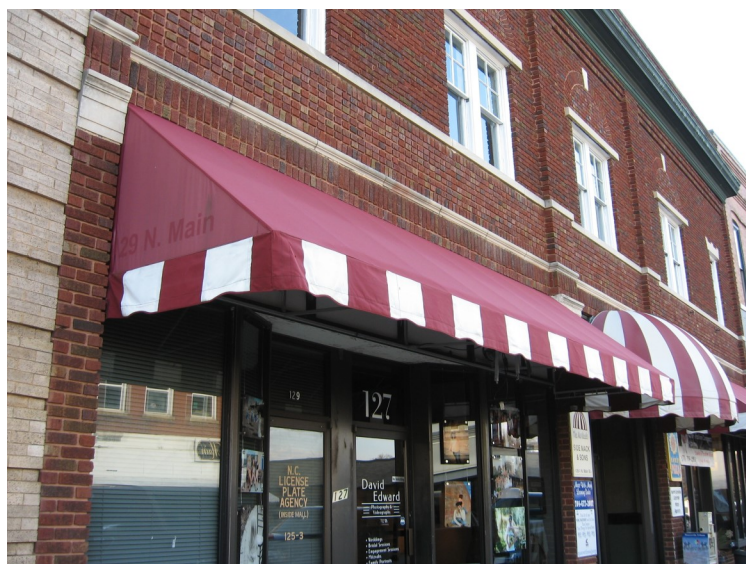
This example of a shed awning is of appropriate placement, materials and color.
