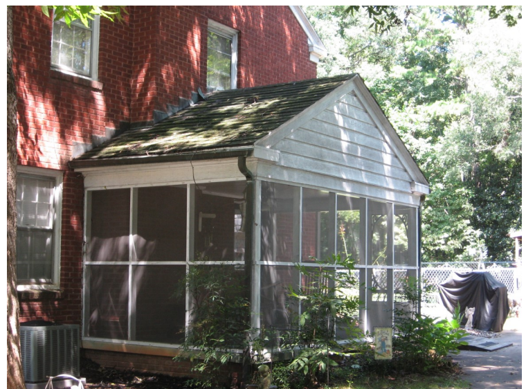
The screening in of porches using minimal framing is appropriate.
