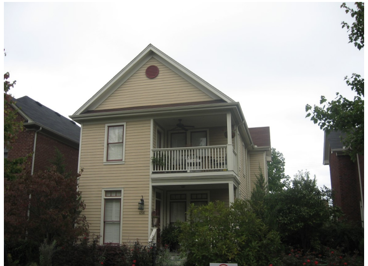
New primary dwellings should have compatible roof forms, materials, fenestration, porches and reflect traditional designs. This infill dwelling has a gable roof, properly sized windows and recessed porches.
