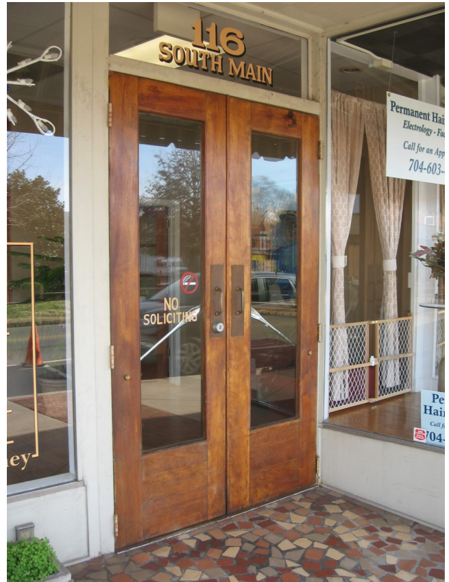
Original double door entrance at this location. .
