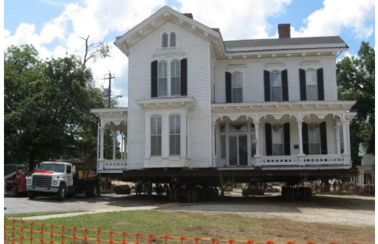
Moving and relocating a historic dwelling such as this house in Raleigh, should be undertaken if demolition would be the only other alternative.
