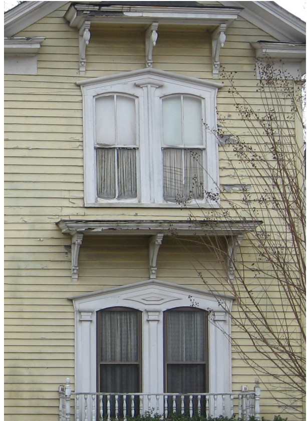
Elongated, narrow windows like these two-over-two, wood-sash examples with pedimented surrounds help characterize this Italianate style dwelling.
