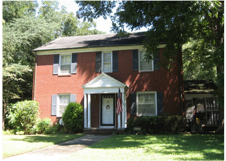
This is an example of a Colonial Revival style dwelling with an original entry porch with square wood columns.
