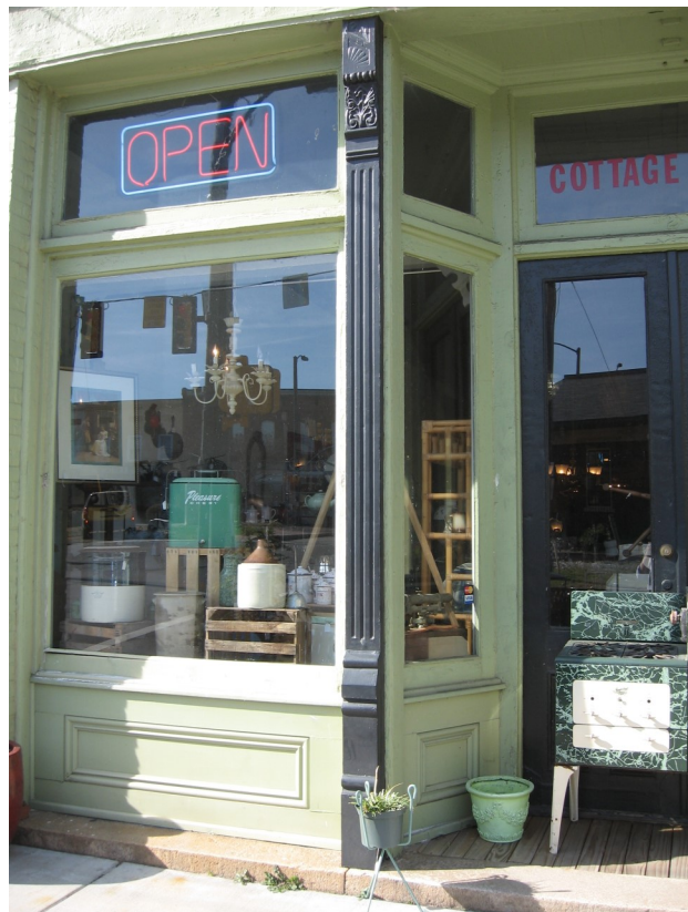
Cast iron pilasters were popular ornamentation and structural elements on turn of the century storefronts.
