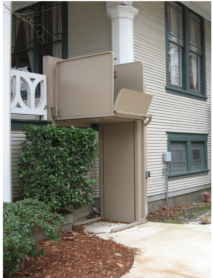
For medical offices and businesses with high demand for ADA compliance, consider the use of chair lifts which can be screened with landscaping and have a minimal impact on the historic
