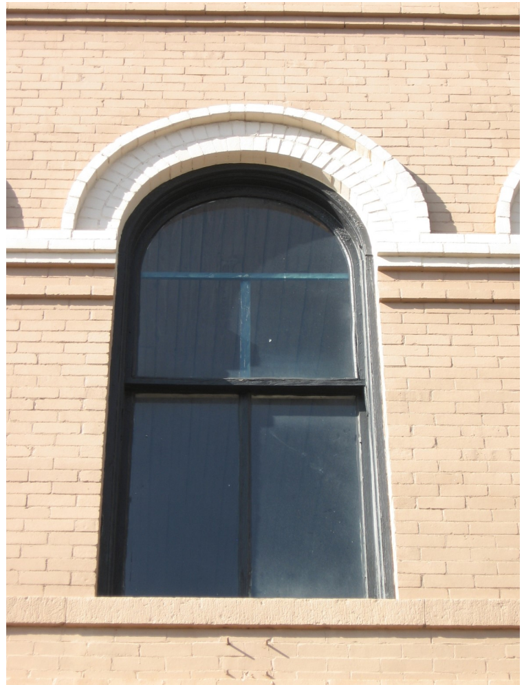
Preserve and maintain original wood sash windows.
