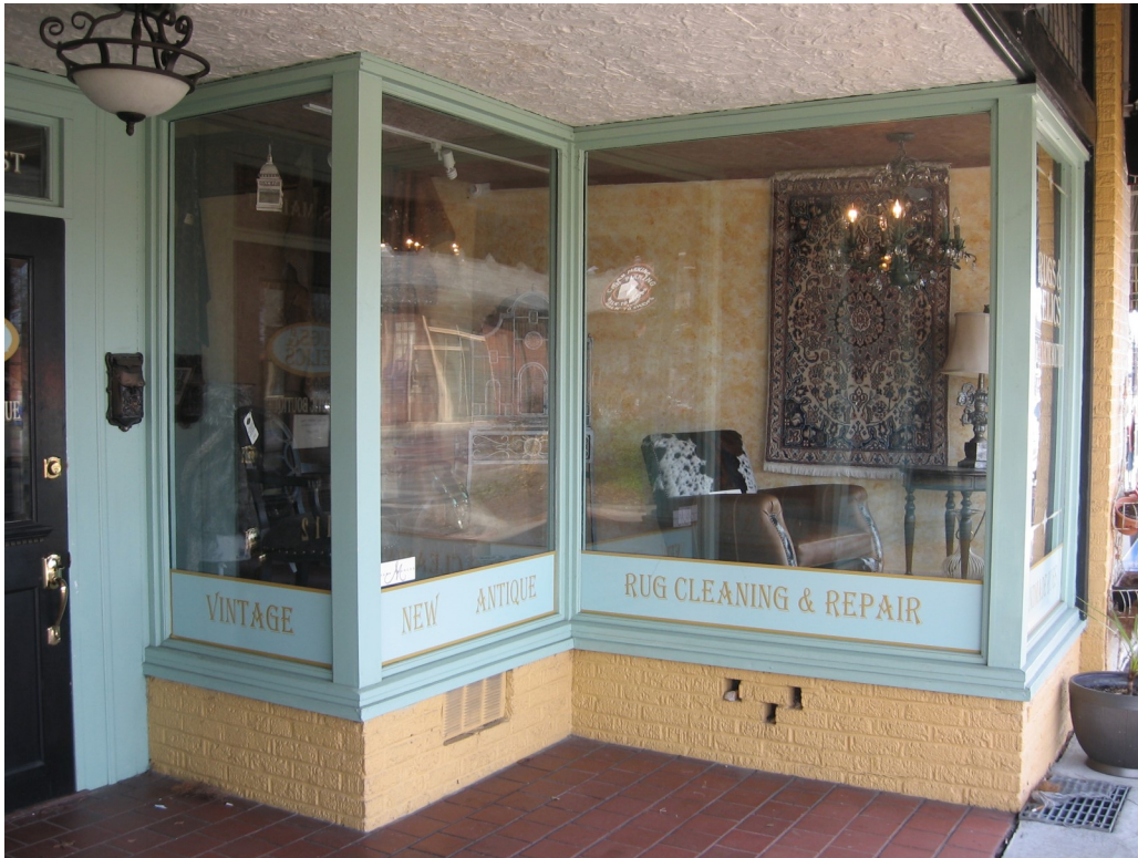
Design guidelines help to ensure the preservation and retention of historic design features such as this original recessed storefront.
