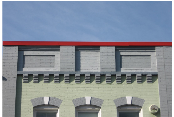
For previously painted masonry walls, paint colors can be used to highlight architectural details.
