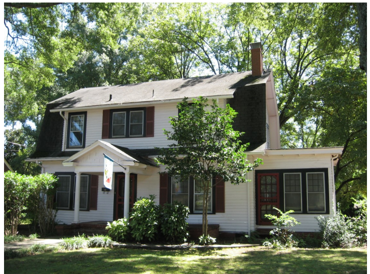
The Dutch Colonial Revival style is distinguished by its gambrel roof form and classical porch columns.
