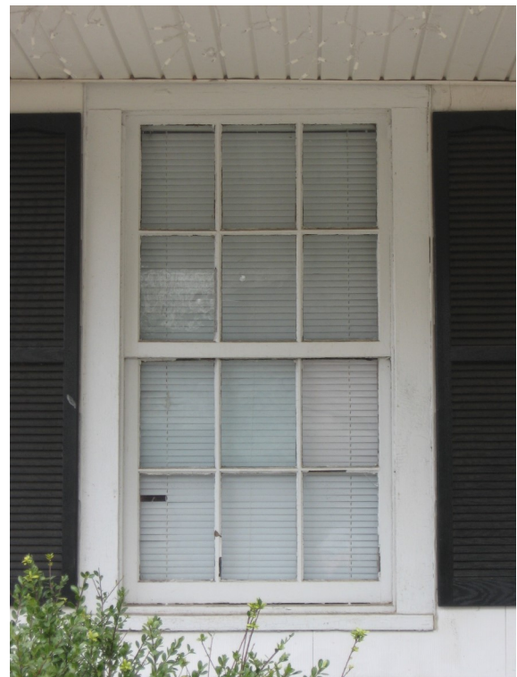
Retain and preserve original wood-sash windows like this six-over-six design.
