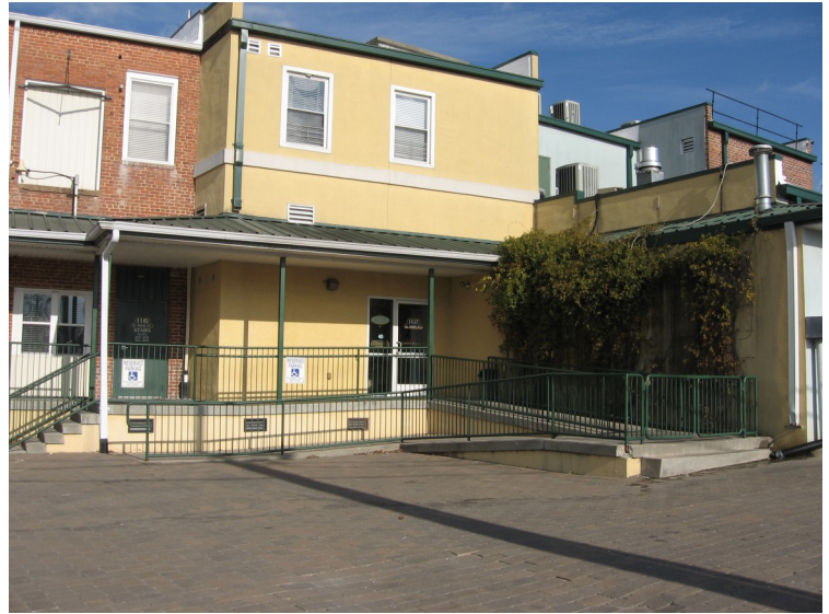
ADA accessibility ramps require staff approval or a COA. These should be sited on rear elevations as in this example.
