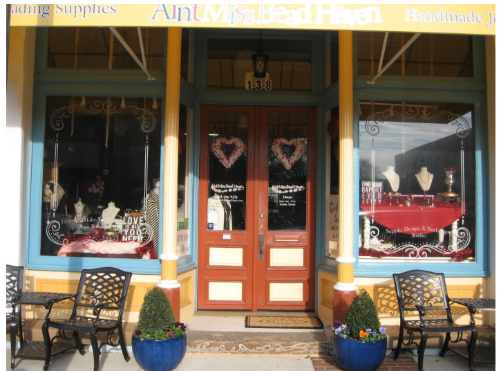
Paint colors can be used to enhance storefront features such as the varying colors on the doors, bulkheads and display windows
