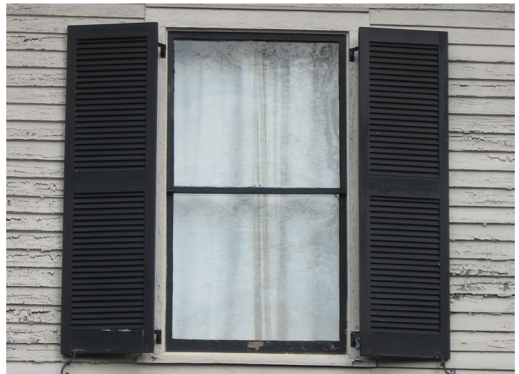
This window has appropriate shutter design and materials.
