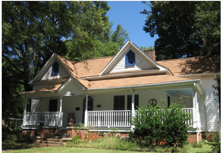
This Folk Victorian dwelling features gable dormers with sawtooth shingles as well as milled porch columns.
