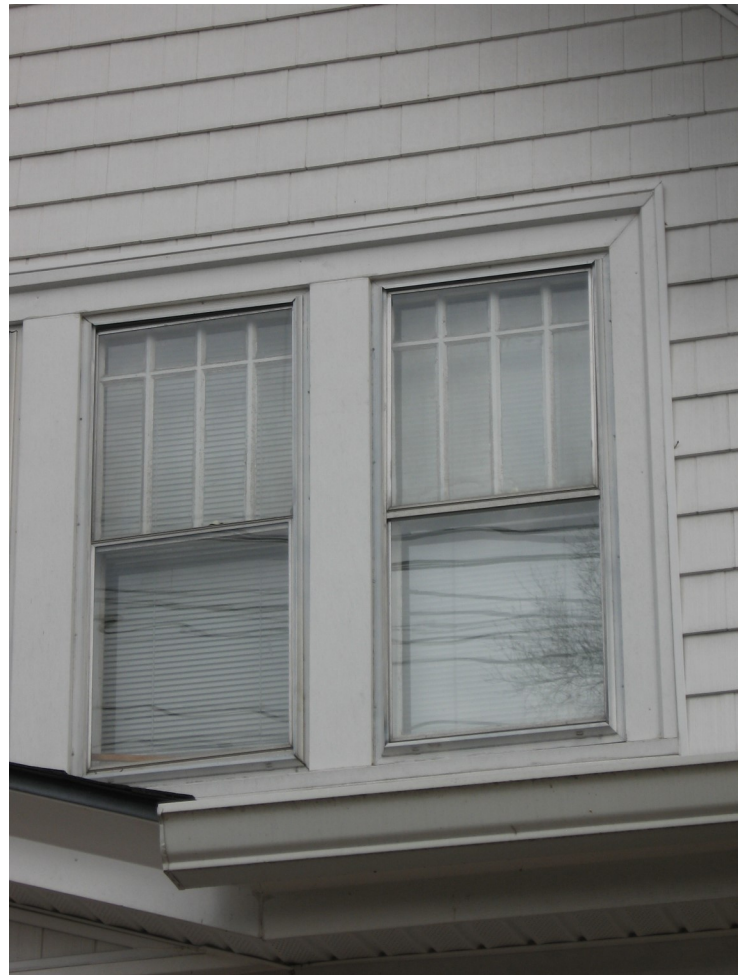
When installing storm windows, choose a full-view design that will not conceal the original windows they covers such as these examples above and below.
