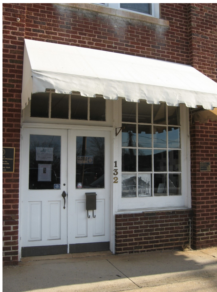
This simple awning is designed to cover both the door and large storefront window.
