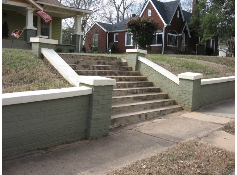
Preserve and maintain original masonry retaining walls.
