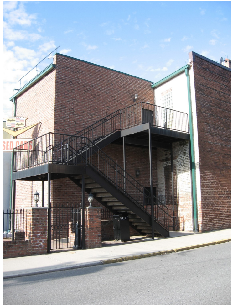
Stairs are appropriately located on the rear elevation of this building.
