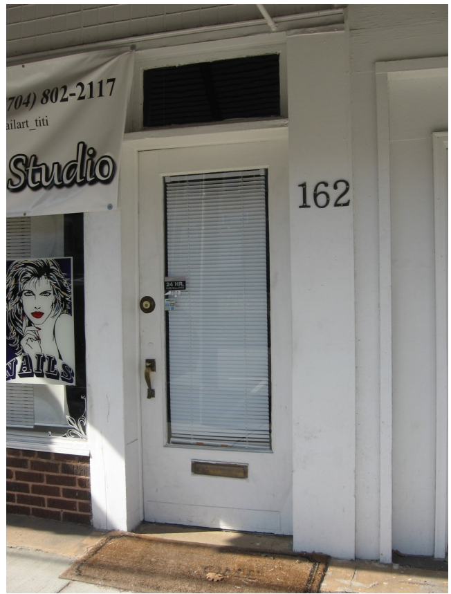
Original single-light door and transom at this building.
