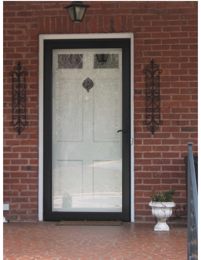
When installing a storm door, choose a full-view design that will not conceal the original door it covers such as the example above.
