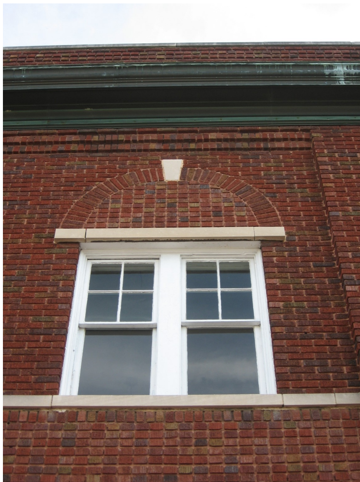
Classical detailing became widely used after 1900 for commercial buildings. This building has sash windows set within an arch with a keystone and decorative brick courses.
