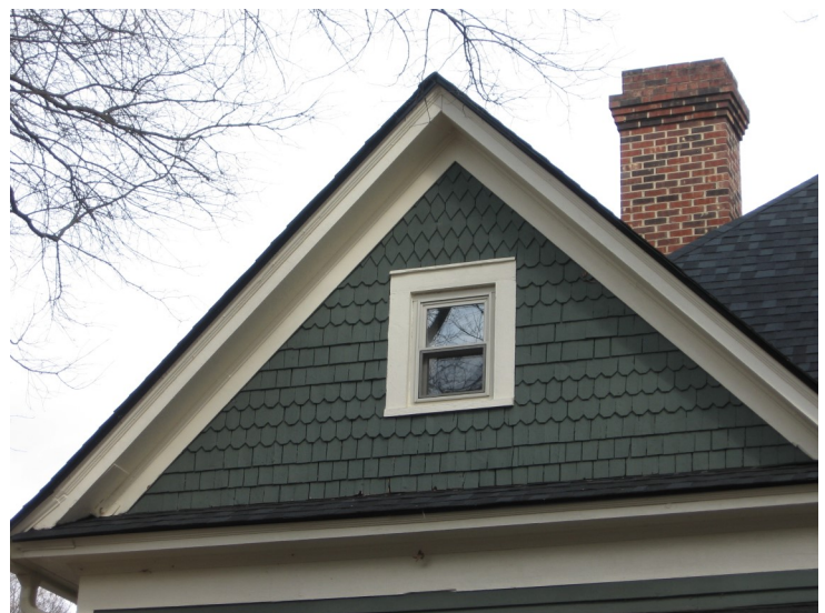
Wood shingles provide texture and should be retained and preserved.
