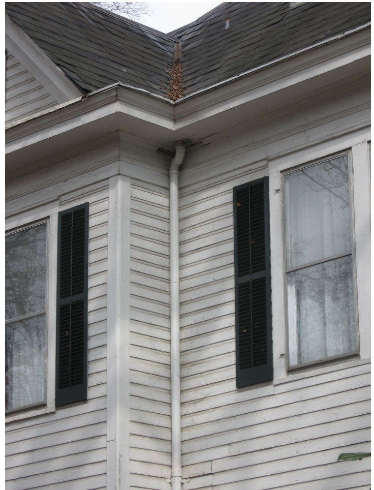
This dwelling retains its original built-in gutter system and round downspouts.
