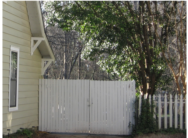
This privacy fence is appropriate in height, materials, and location. It is properly recessed to the rear corner of the dwelling.
