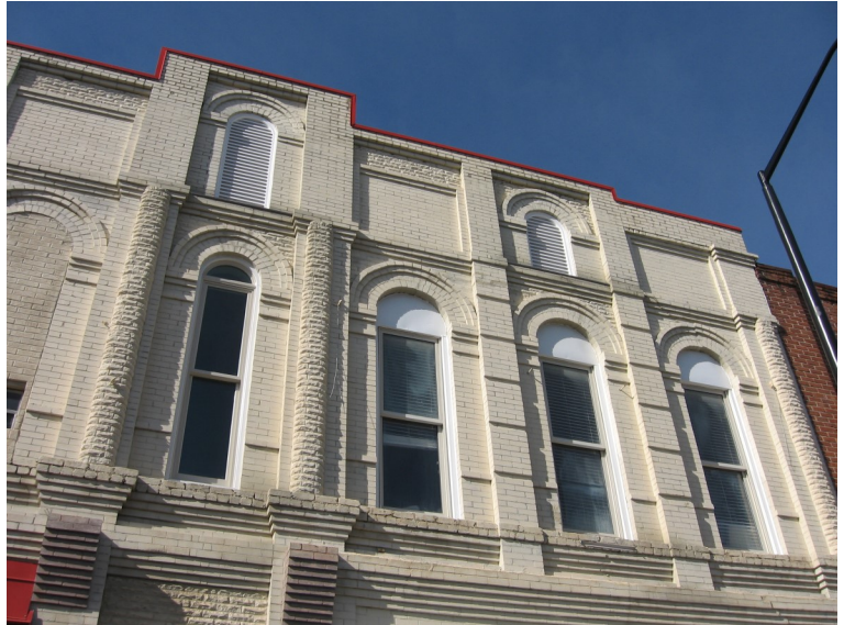
The upper façade of this commercial building has arched sash windows emphasized by pilasters.
