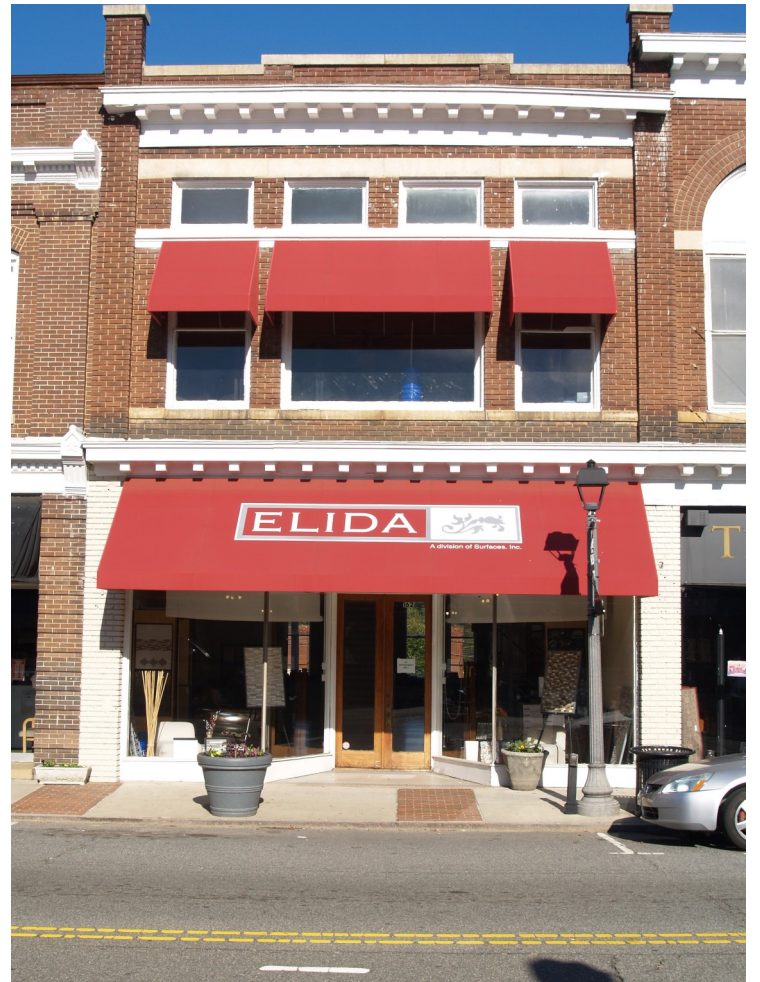
Two-part commercial blocks are at least two-stories in height and have separate storefronts and upper façades.
