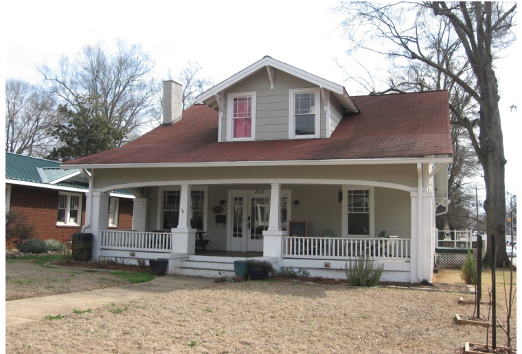
This Bungalow dwelling has an original full-width porch with tapered wood posts on brick piers and a prominent gable dormer at the roofline.
