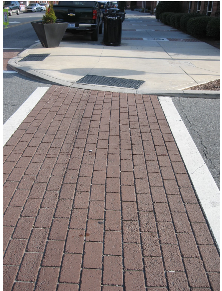
ADA compliant crosswalks have been incorporated into city streets and sidewalks in downtown Mooresville.
