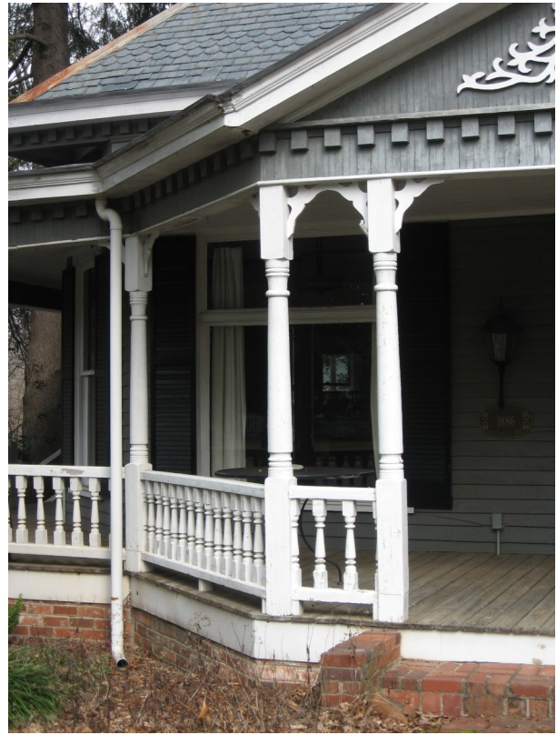
Milled wood porch elements are character-defining features on Victorian-period dwellings.
