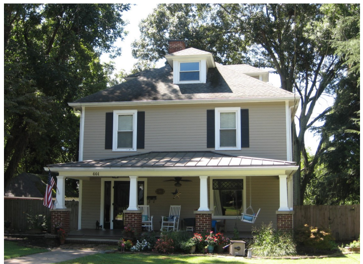
The American Foursquare plan features a full-width porch and a hipped dormer at the roofline.
