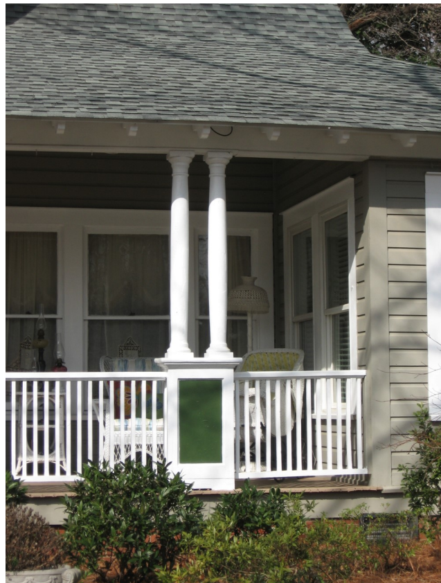
After 1900, classical columns such as Tuscan designs were popular for porches.
