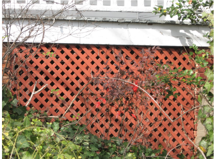
The use of lattice panels between brick pier foundations is appropriate and encouraged.
