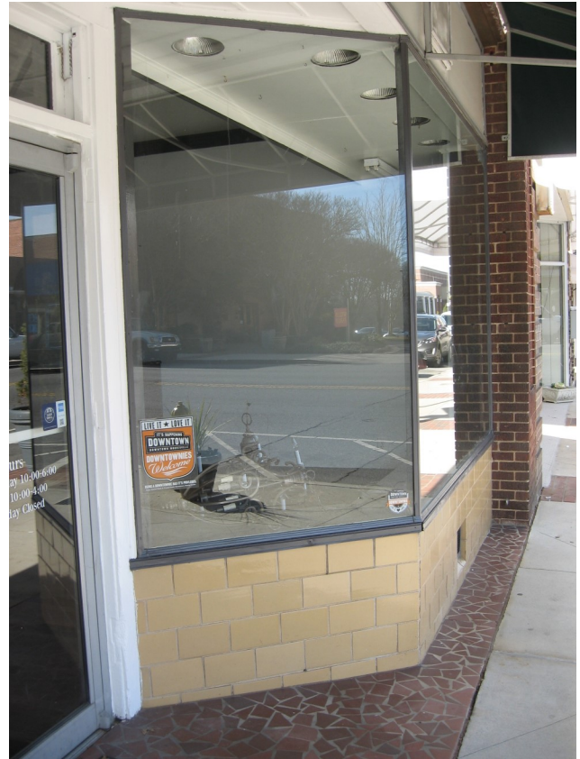
The use of glazed tile was popular for bulkheads during the 1930s and 1940s.
