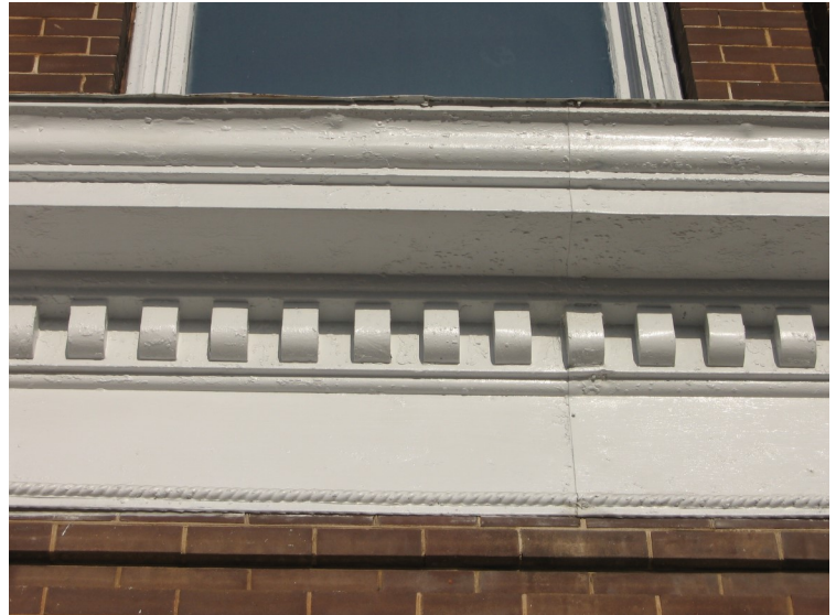
Example of a well preserved and maintained sheet metal cornice.
