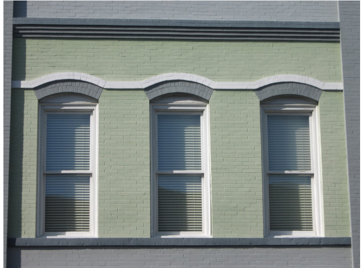
One-over-one wood sash windows are the most common historic designs in the downtown area .
