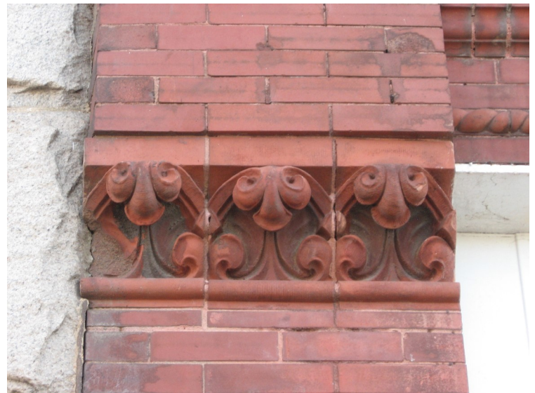
A few examples of decorative terra cotta are visible downtown such as this floral capital.
