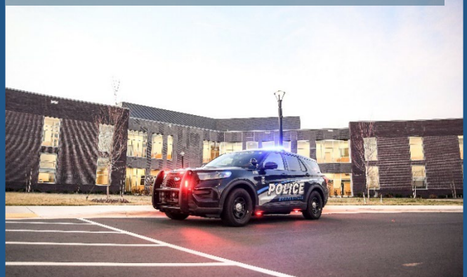
Mooresville Police Department Headquarters
