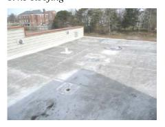
The walk out roof is a white Duro-Last membrane which was would assume was used at the roof above the second floor.
