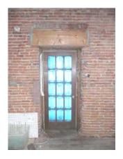
The south entry door at grade is a 3'-0" x 7'-0" insulated glass metal storefront door in good condition.
