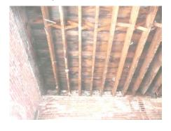
The roof framing, as estimated from below, is 2"x9 7/8" joists at ~12" on center. The roof deck is wood planking of undetermined thickness. It is not known whether another layer of decking was put down associated with a new roof. The roof joists appear to be in fair condition.
