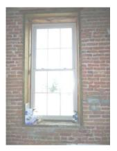
The north windows are insulated double hung with prefinished metal clad exterior and interior in fair condition and measure 33" wide and 73" high.
