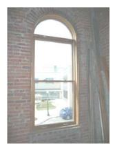
The south windows are insulated double hung with a prefinished metal clad exterior and unfinished pine interior that are in fair condition. They measure 36" wide and 73" high.
