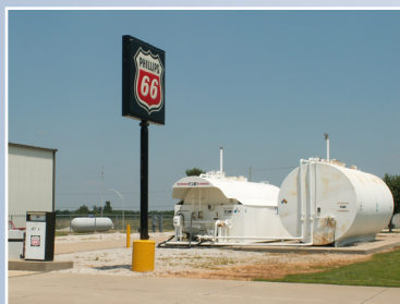
100LL & Jet A Fuel Facilities (airside)
