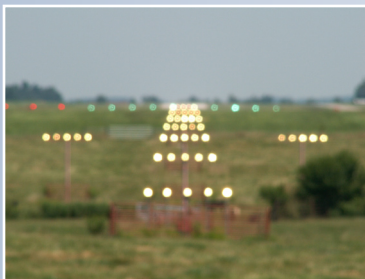
Runway 36 MALSF Approach Lighting System and PAPI-4L Visual Approach Aid
