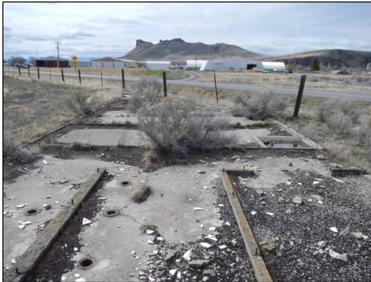
Photograph 6. Block 71 partial latrine slab [REDACTED] (view to southwest)
