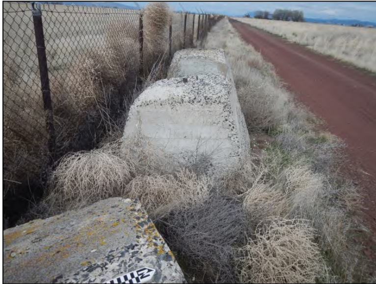
Photograph 4. TLSC Guard Tower Footings (view to northwest)
