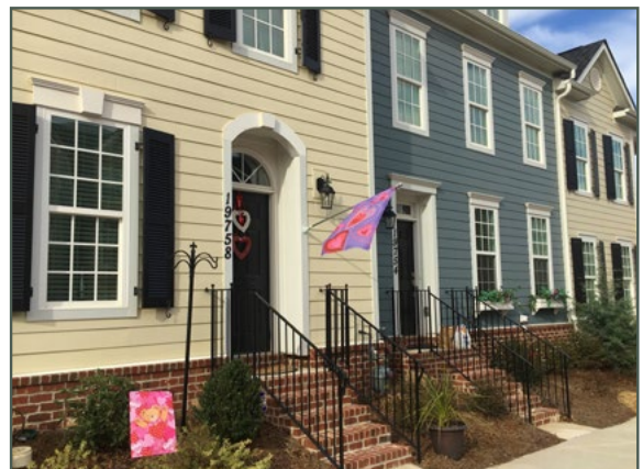
Brick steps and foundation with rowlock water mark and iron railing where applicable.
