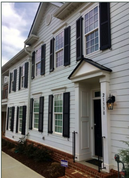
Recessed front door with pediments with operable shutters, with hinges and shutter dogs.
