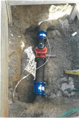
(Installation of new gate valve)
