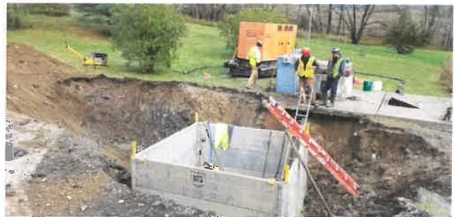
(Halpin Road Pump Station repair.)
