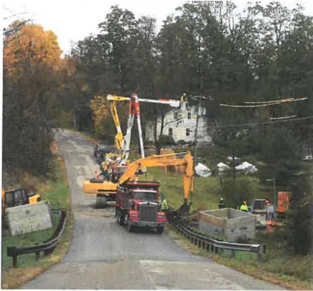
(Halpin Road Pump Station repair.)
