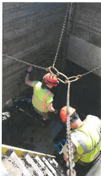
(Repairing hole in water main with stainless steel wrap.)
