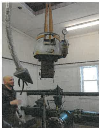
Removing the pump and motor at Palmer Springs and the scored pump shaft.
