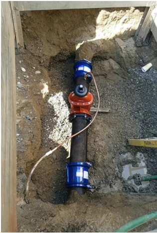
(Installation of new gate valve)
