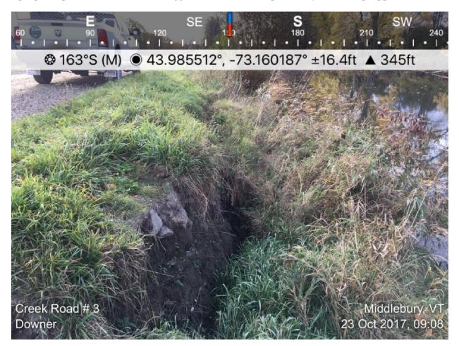
The deep ditch on the east side of the road encourages saturation of the road embankment. ►
