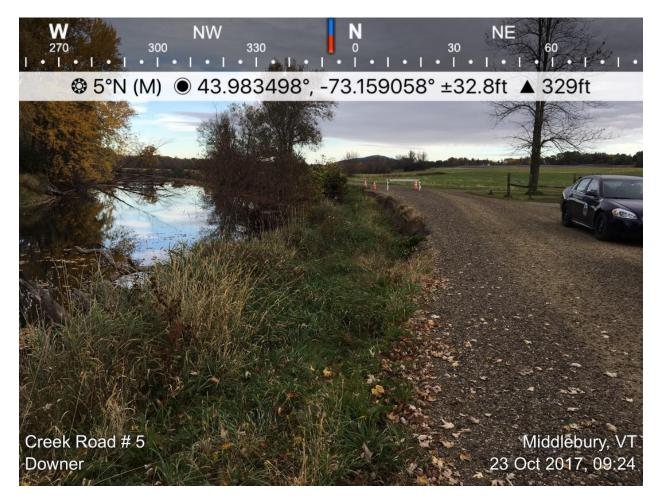
This section of bank slipped downward about 2 feet. The slightly back sloping of the grassed area suggests a rotational failure occurred; probably resulting from saturated soils coincident with erosion at the bank toe.
