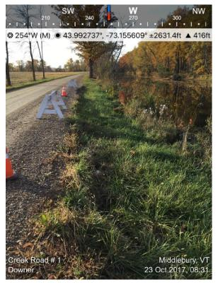
◄ Grassed section of the bank rotated downward about 8 inches. Note that there are no trees on this section. The shoulder of the road did not move.
