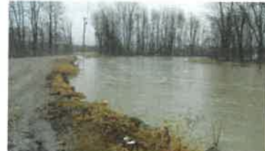
Three Mile Bridge Road & Middlebury River
