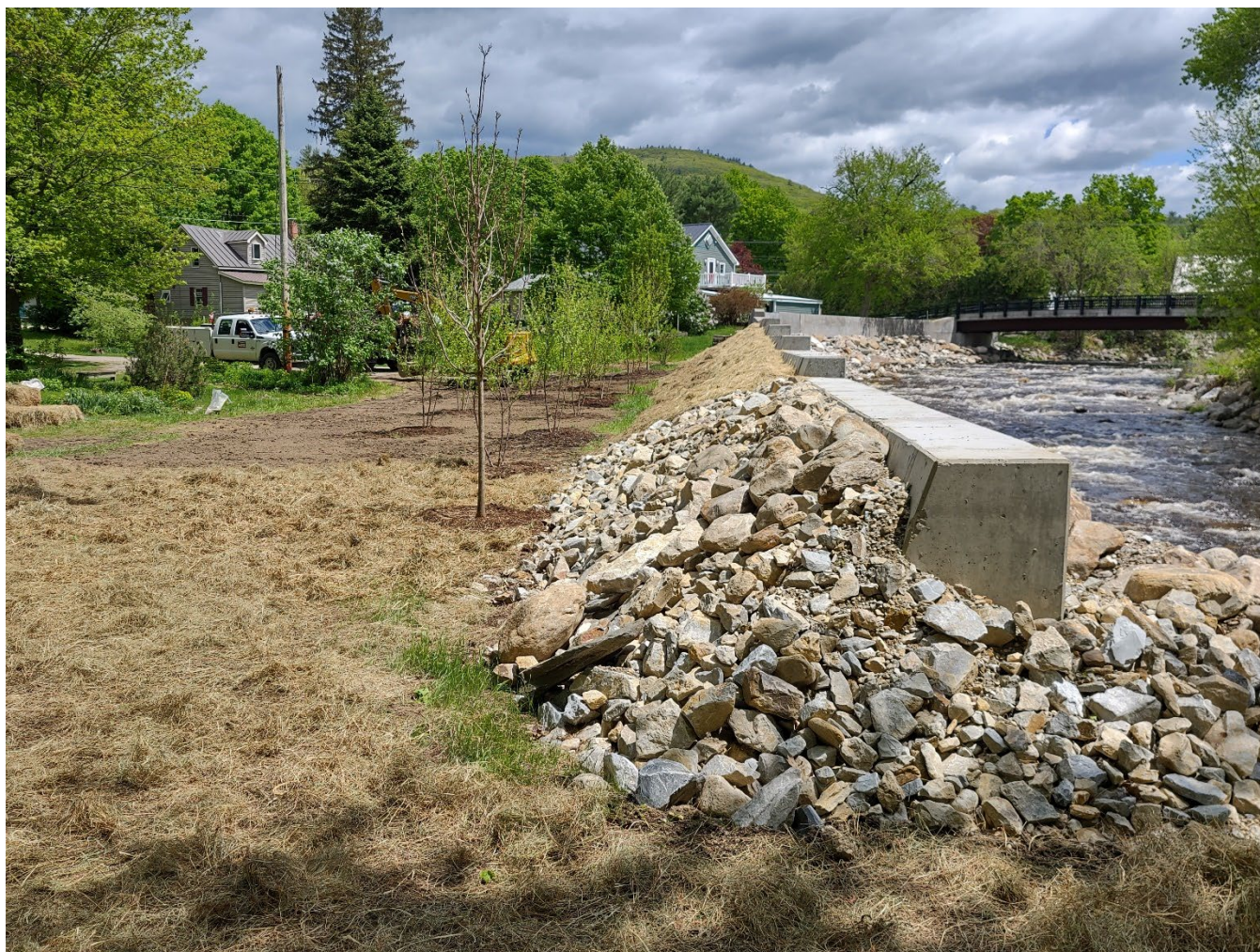
Figure 2: Restoration underway at the new flood wall, planted maple visible at the base of the stone slope.
