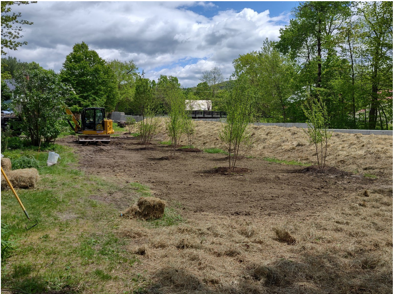
Figure 1: Work underway to restore disturbed area at the new flood wall. Earthen slope behind new flood wall has been seeded and mulched. River birch clusters planted along the base of the earthen slope.
