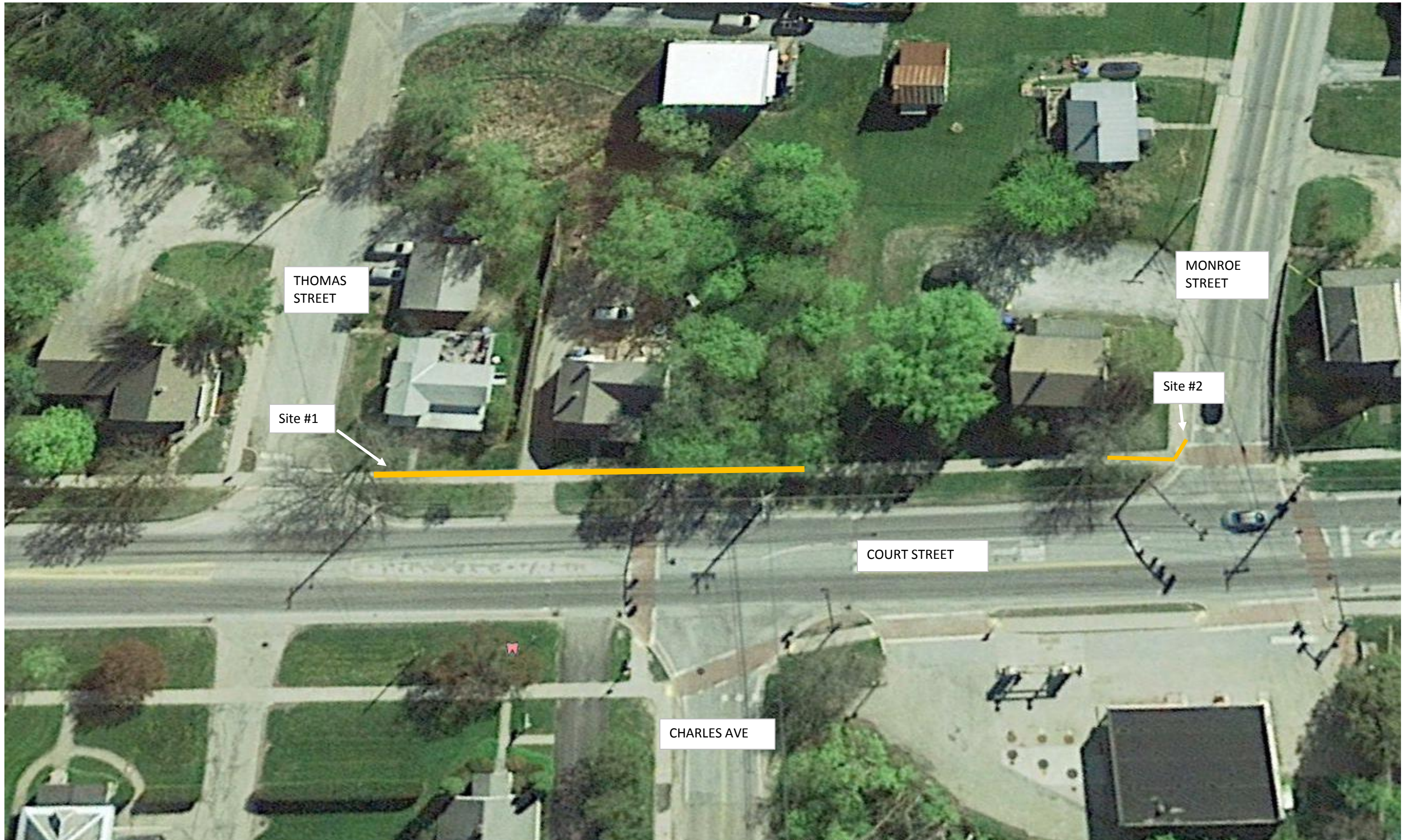
COURT STREET (RT 7)
