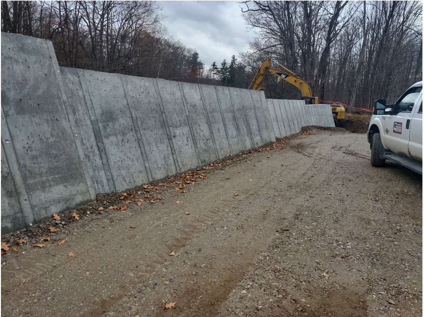
Figure 1: View of completed backfill behind new flood wall extension, only final section remains once concrete has cured enough to be backfilled.
