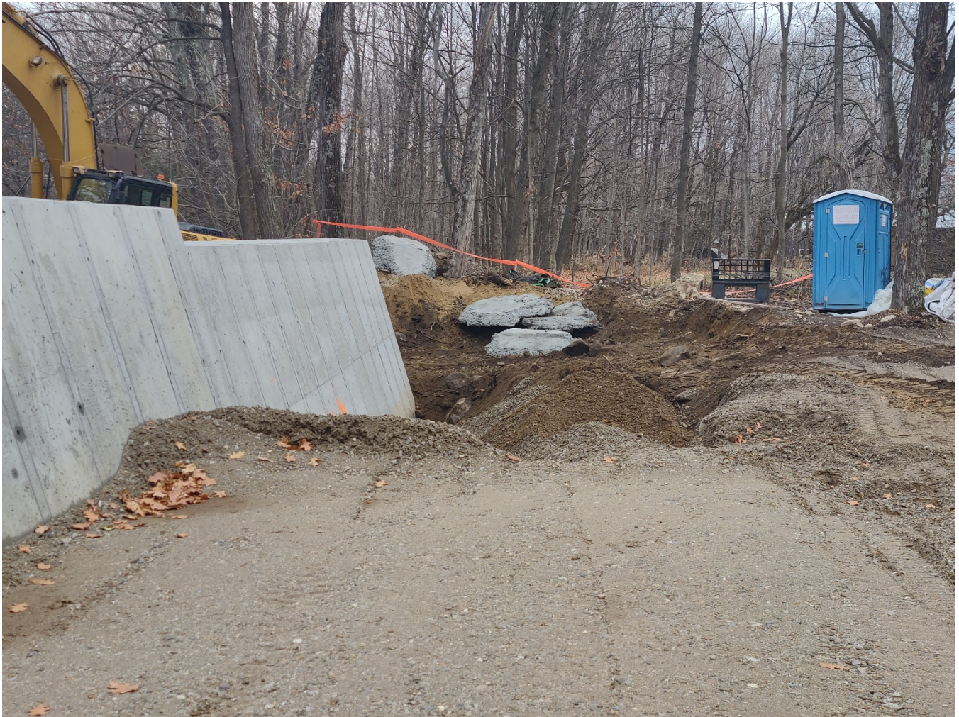
Figure 2: Concrete “pads” (visible in the background) and other miscellaneous trash being removed from the river prior to removing access road.
