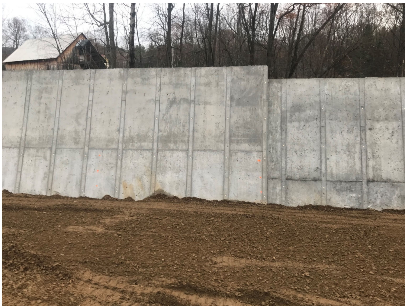
Figure 2: Filling behind wall with gravelly material.
