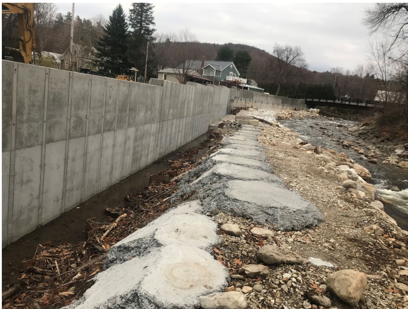
Figure 3: Concrete pads to be removed from site when access road material will be moved to the wall to protect new foundation.
