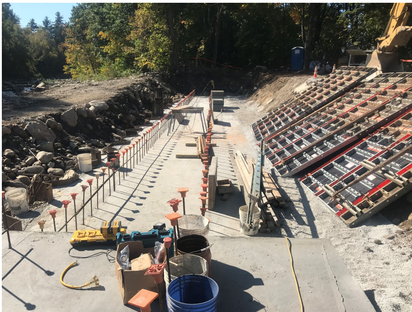
Figure 2: Curing foundation with rebar for flood wall.
