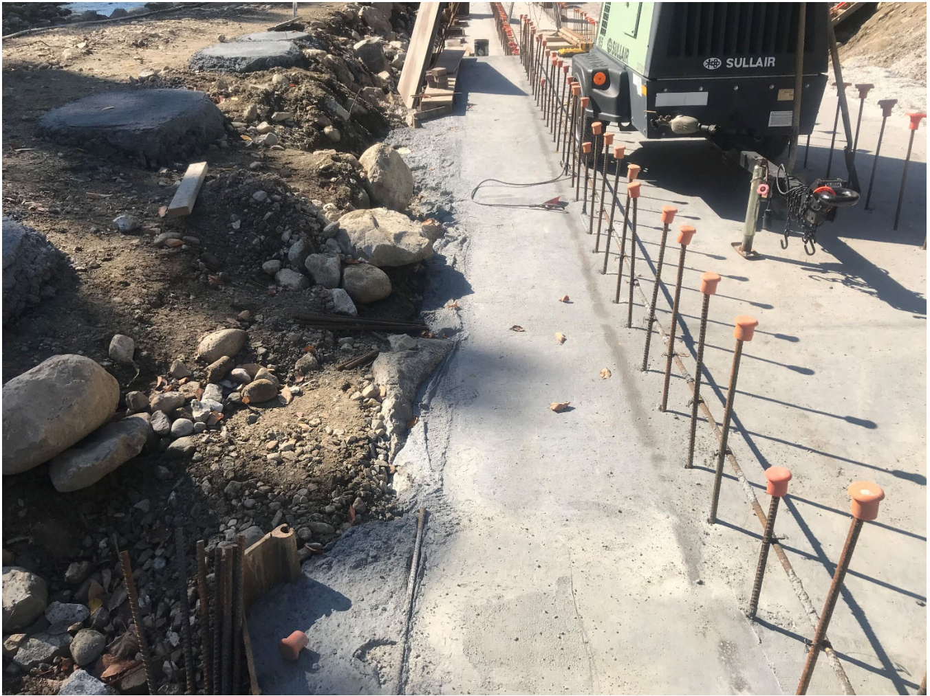
Figure 3: Gap in sheeting where the wall is pinned to existing concrete and boulders.
