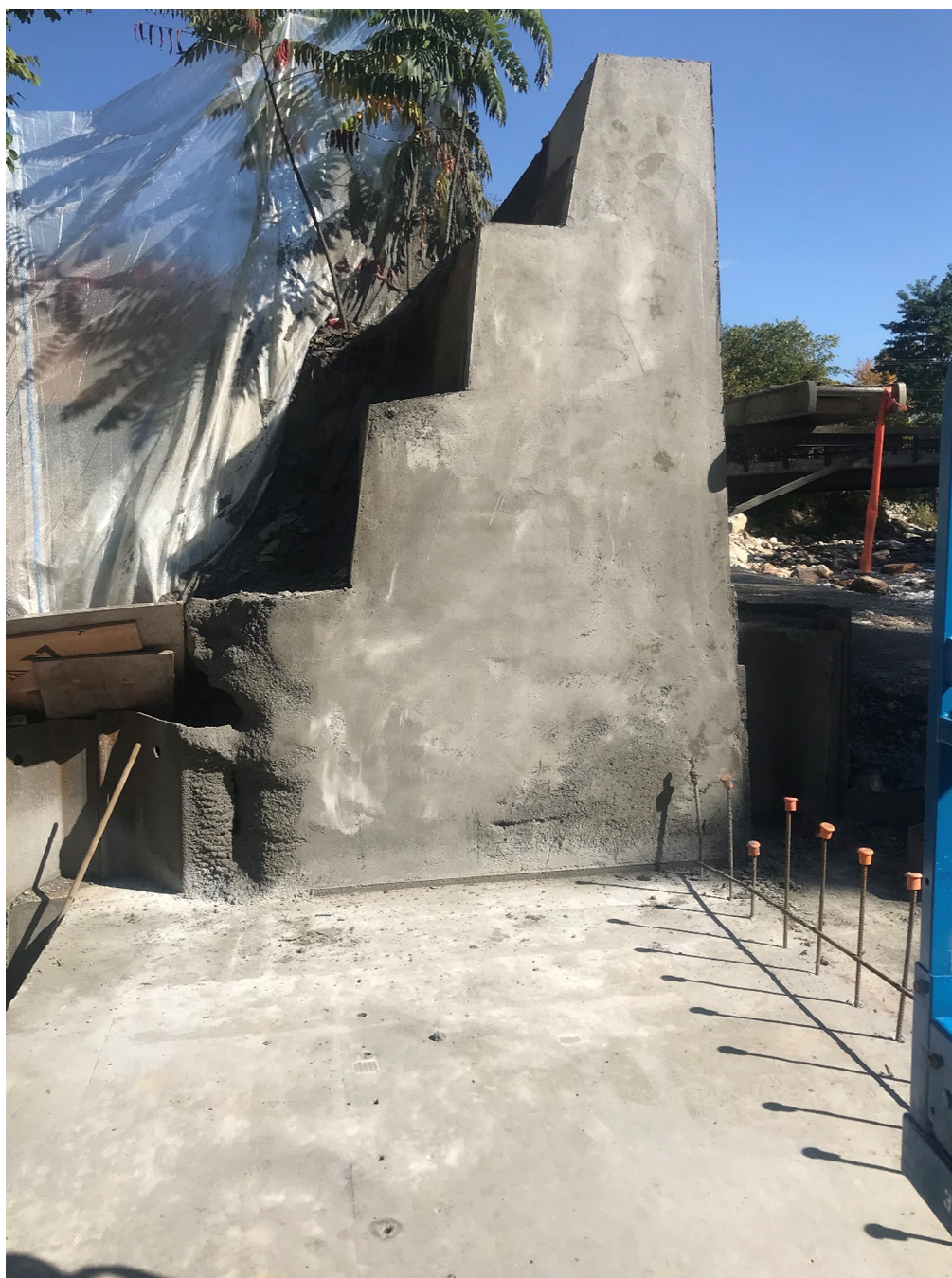
Figure 1: End of existing wall smoothed for connection to proposed wall via expansion joint.
