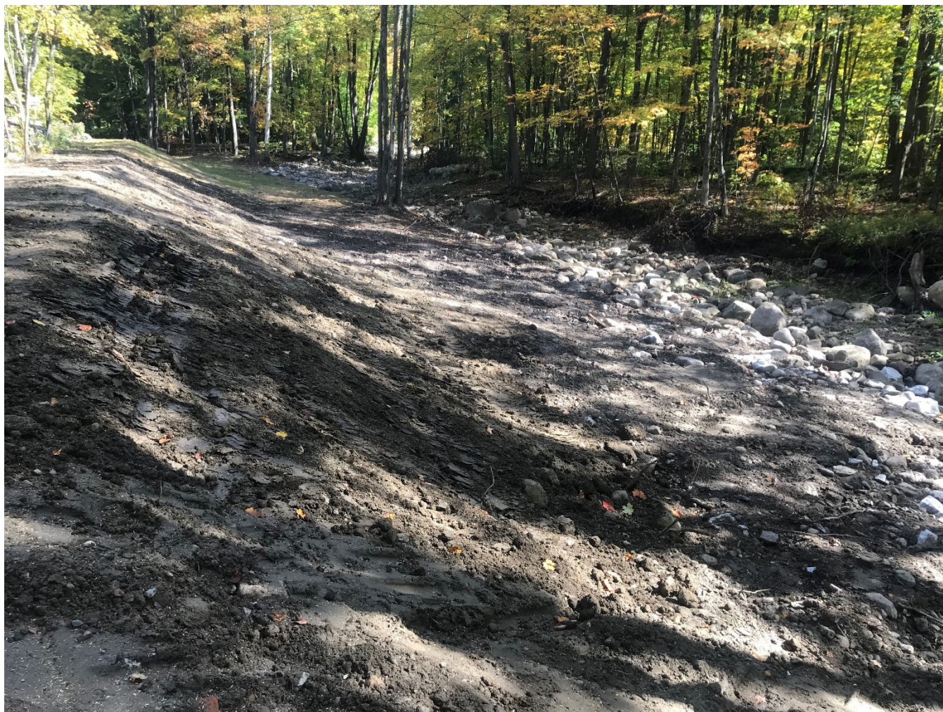
Figure 4: Completed stone armor with soil and seeding at the upstream site awaiting mulch.
