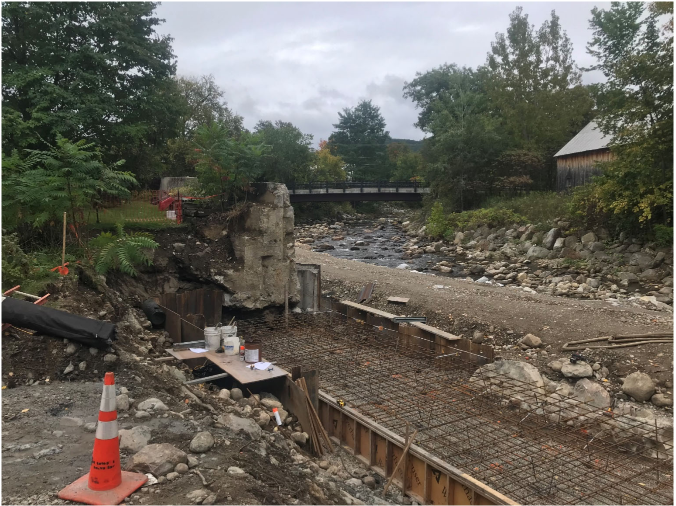
Figure 2: Rebar installation and forming in preparation of concrete pouring in upstream portion of proposed flood wall.
