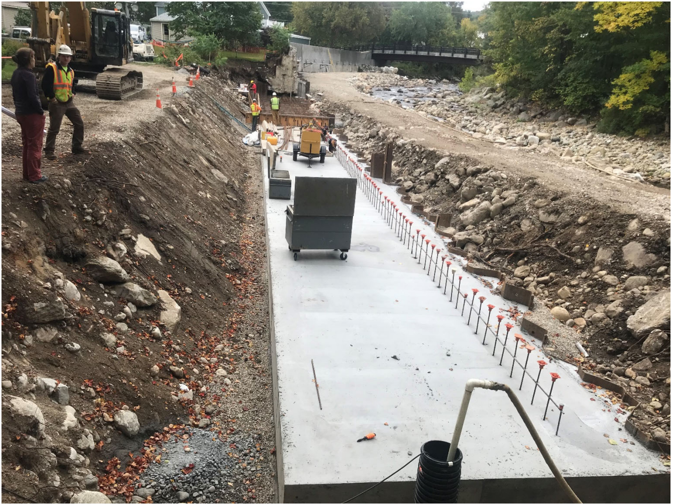
Figure 4: Overview of proposed flood wall under construction.
