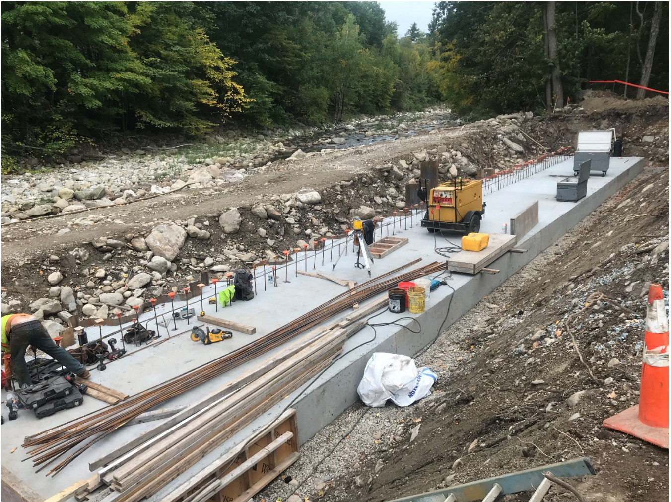
Figure 3: Foundation of the downstream portion of the proposed floodwall.
