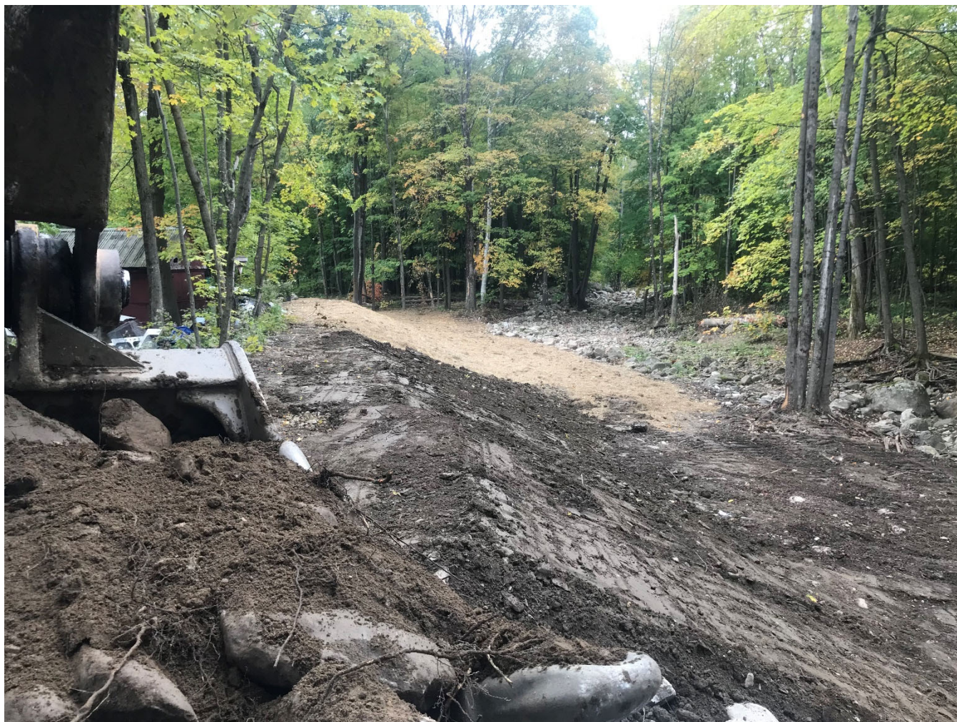
Figure 1: Stone armor and grubbing continues near the Welch property.
