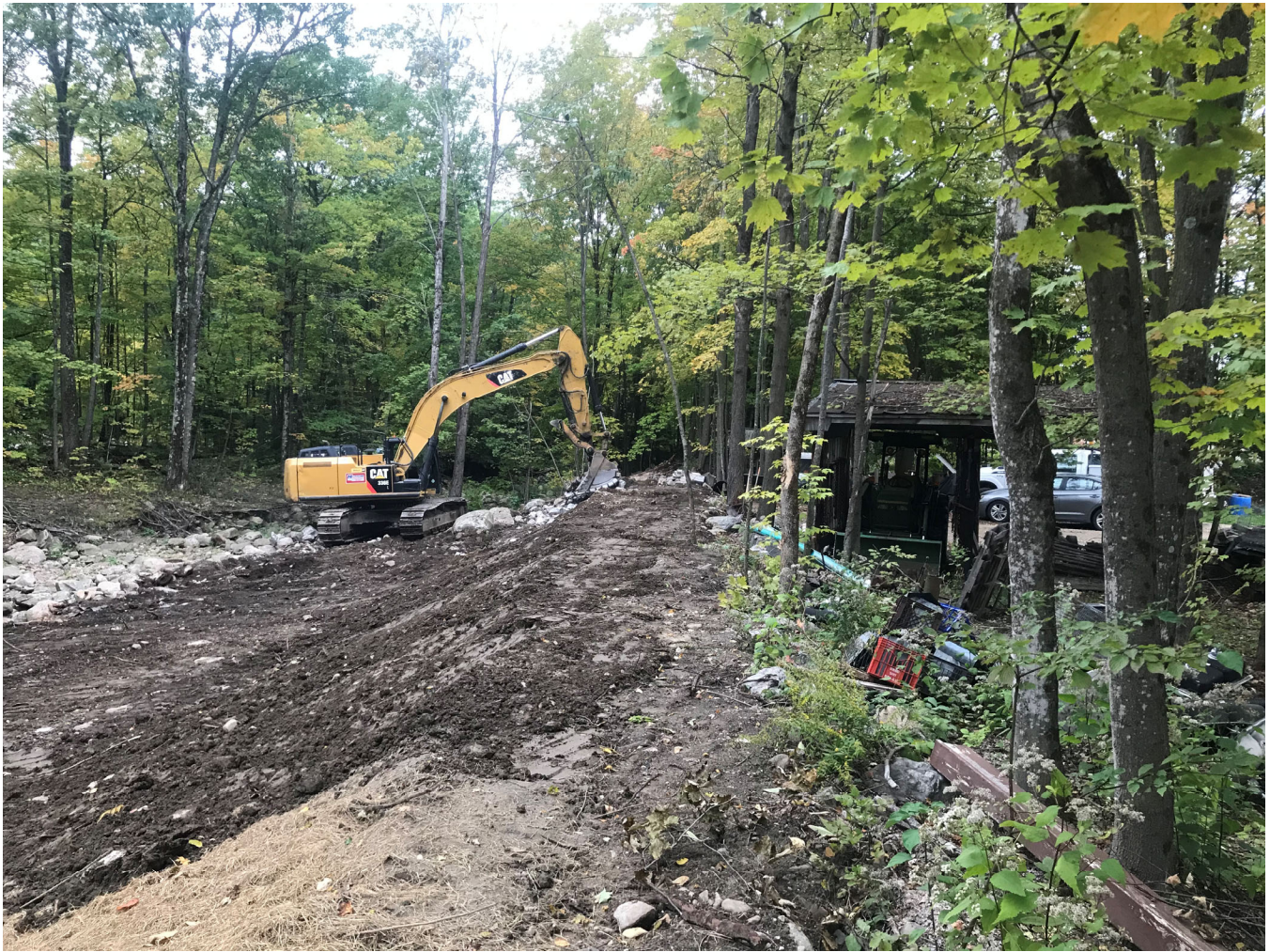
Figure 5: Stone armor installation near the Welch property.
