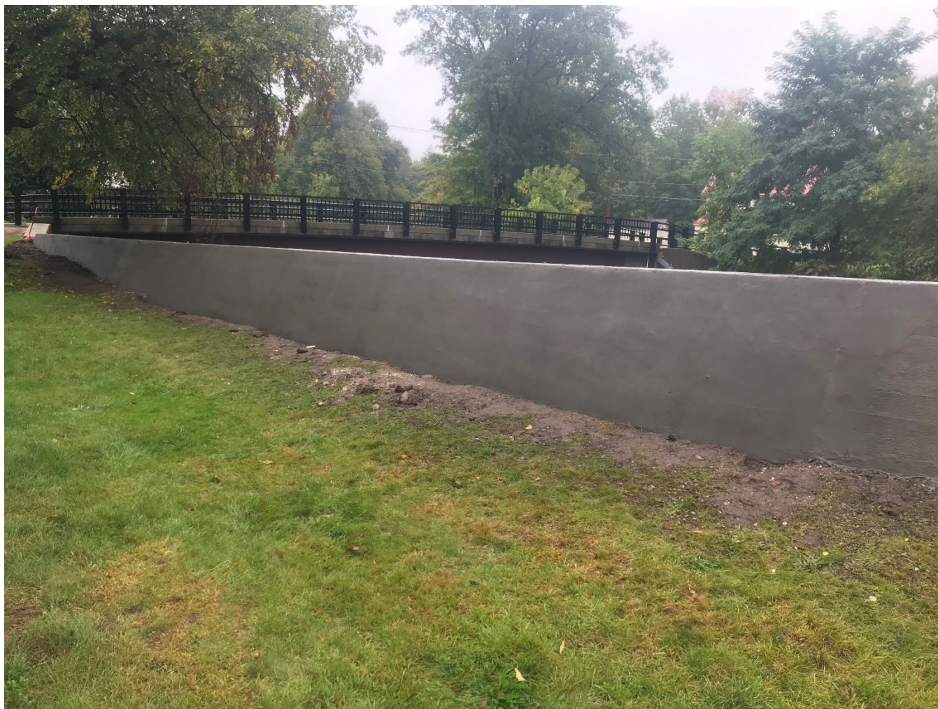
Figure 3: Skim coating repair on the back of the flood wall.
