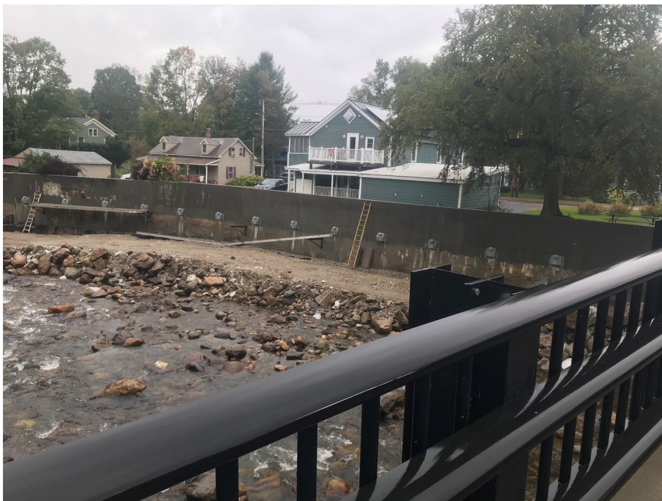
Figure 2: Repair of the existing floodwall nearing completion.
