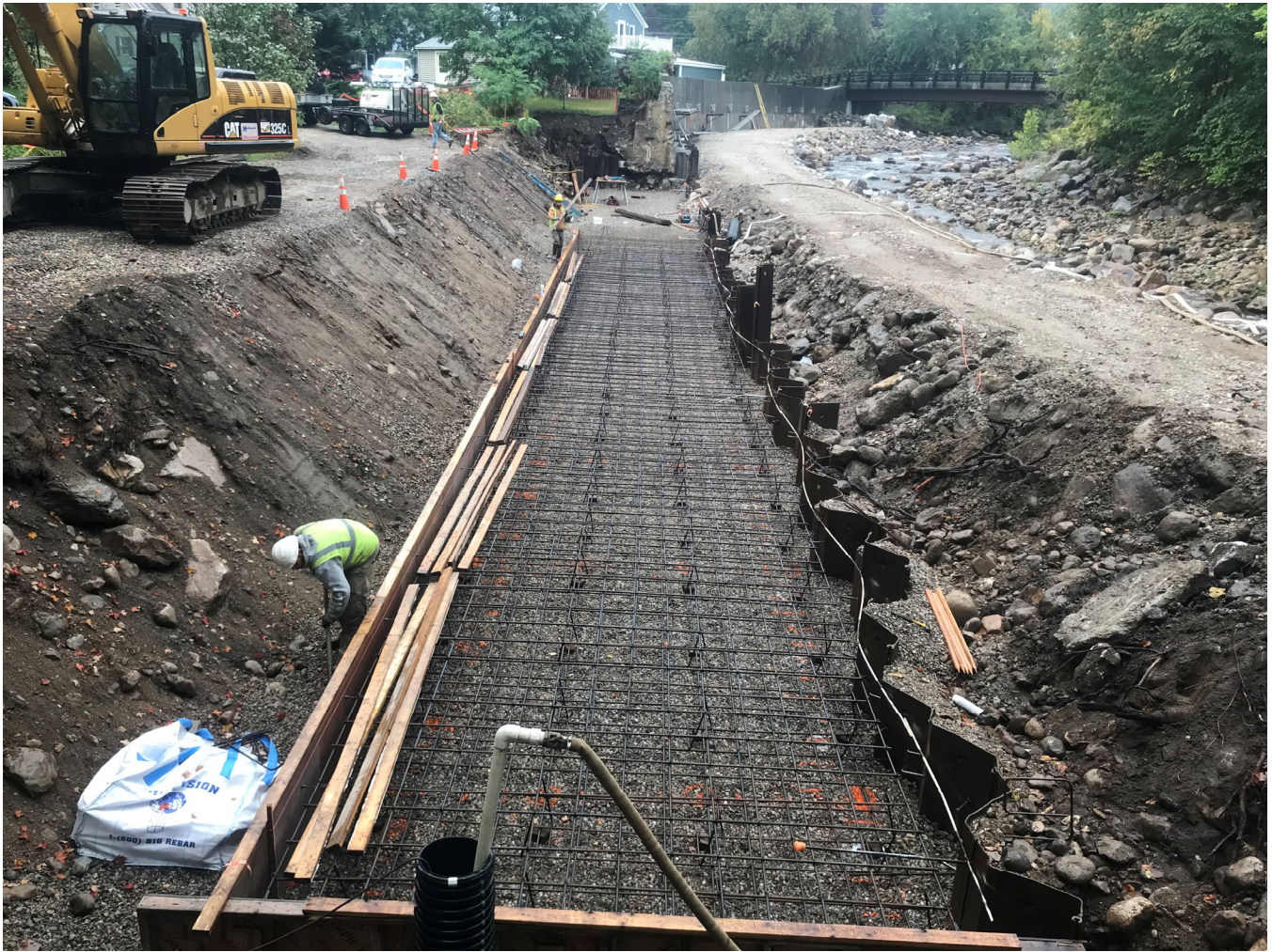
Figure 5: Rebar installation and forming in preparation of concrete pouring in downstream portion of proposed flood wall.
