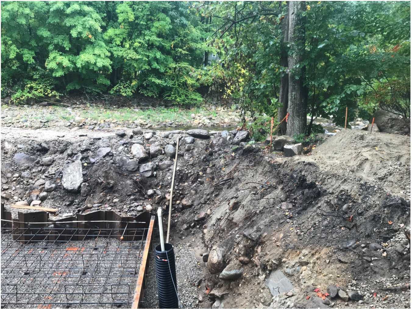
Figure 4: Proposed gap between flood wall (white steel bar with cap) and tree to be 13.5 feet.
