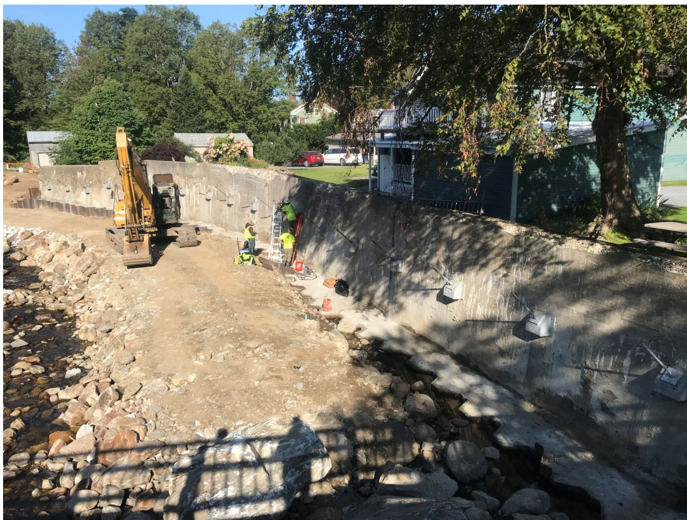
Figure 2: Ground anchor testing.
