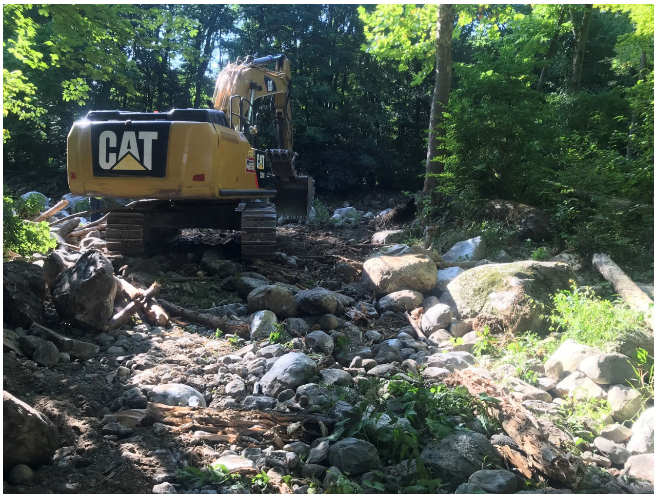
Figure 4: Cleaned out upstream flood chute.
