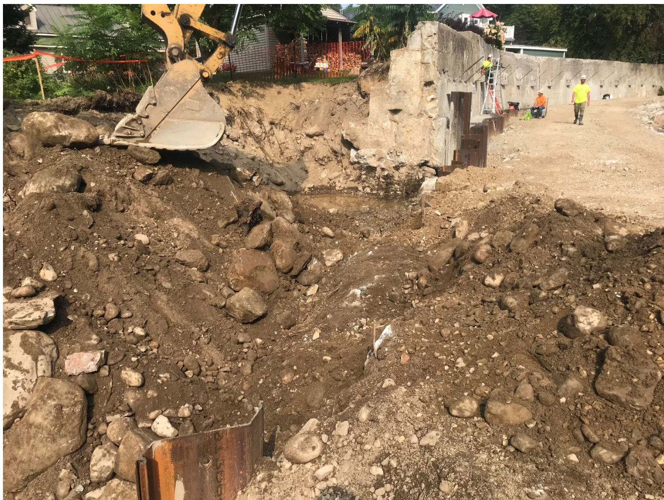
Figure 5: Sheet piling installed for new flood wall section, minus the area with concrete that cannot be excavated.
