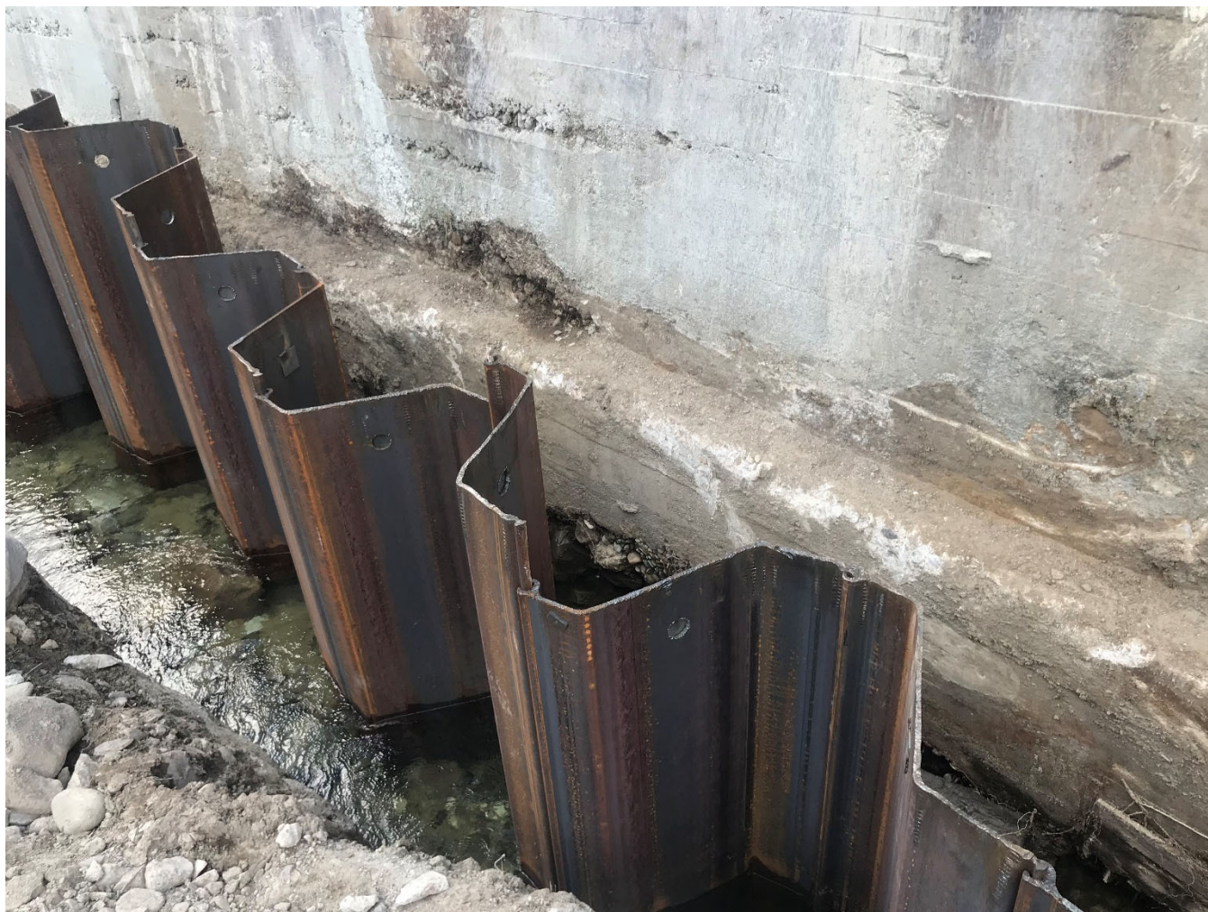
Figure 2: Close-up of driven sheeting.
