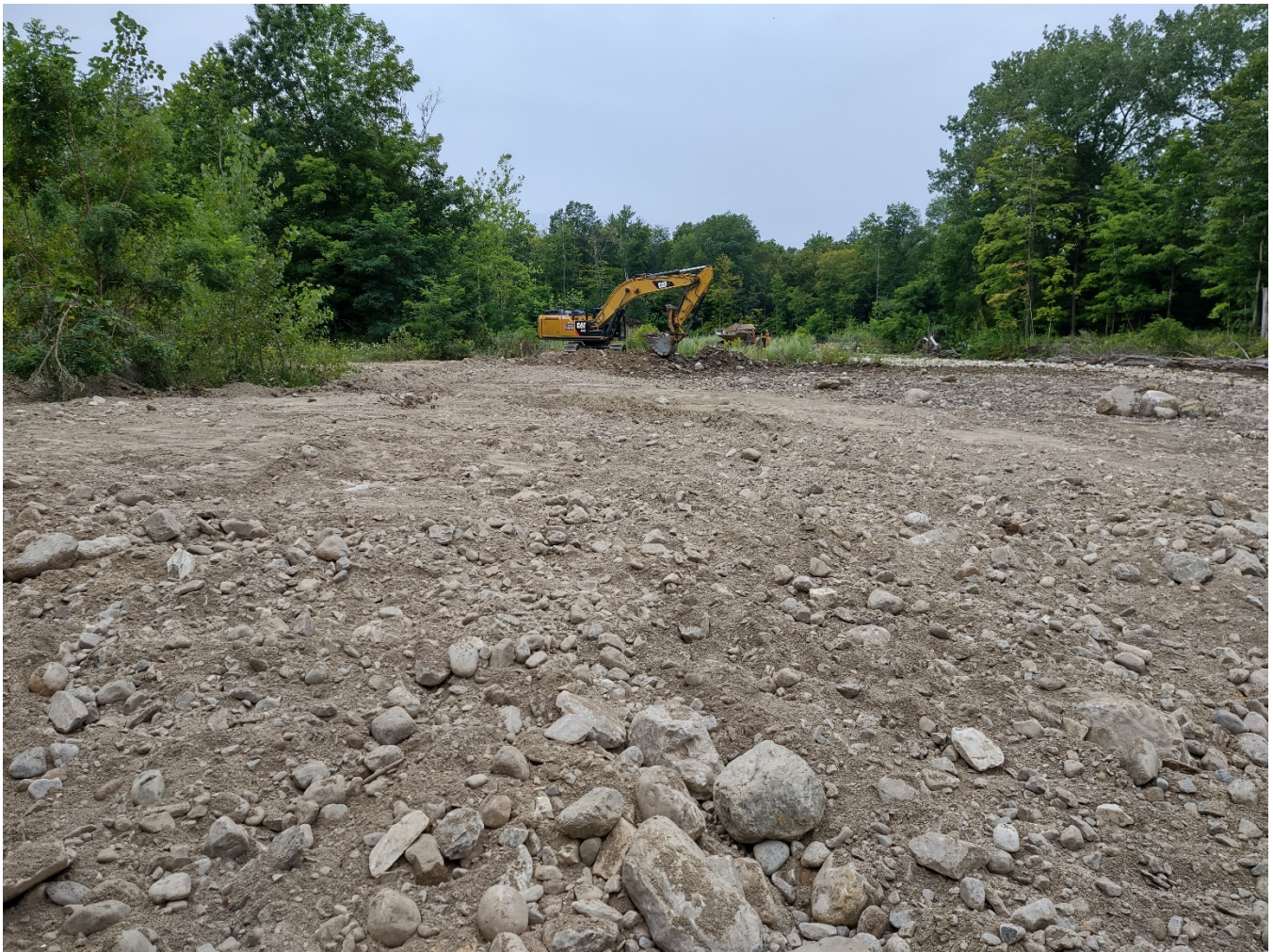
Figure 1: Gravel removal underway at Sediment Bar F.
