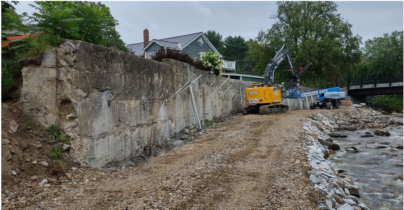
Figure 4: ground anchor installation underway at the Grist Mill Road Floodwall.
