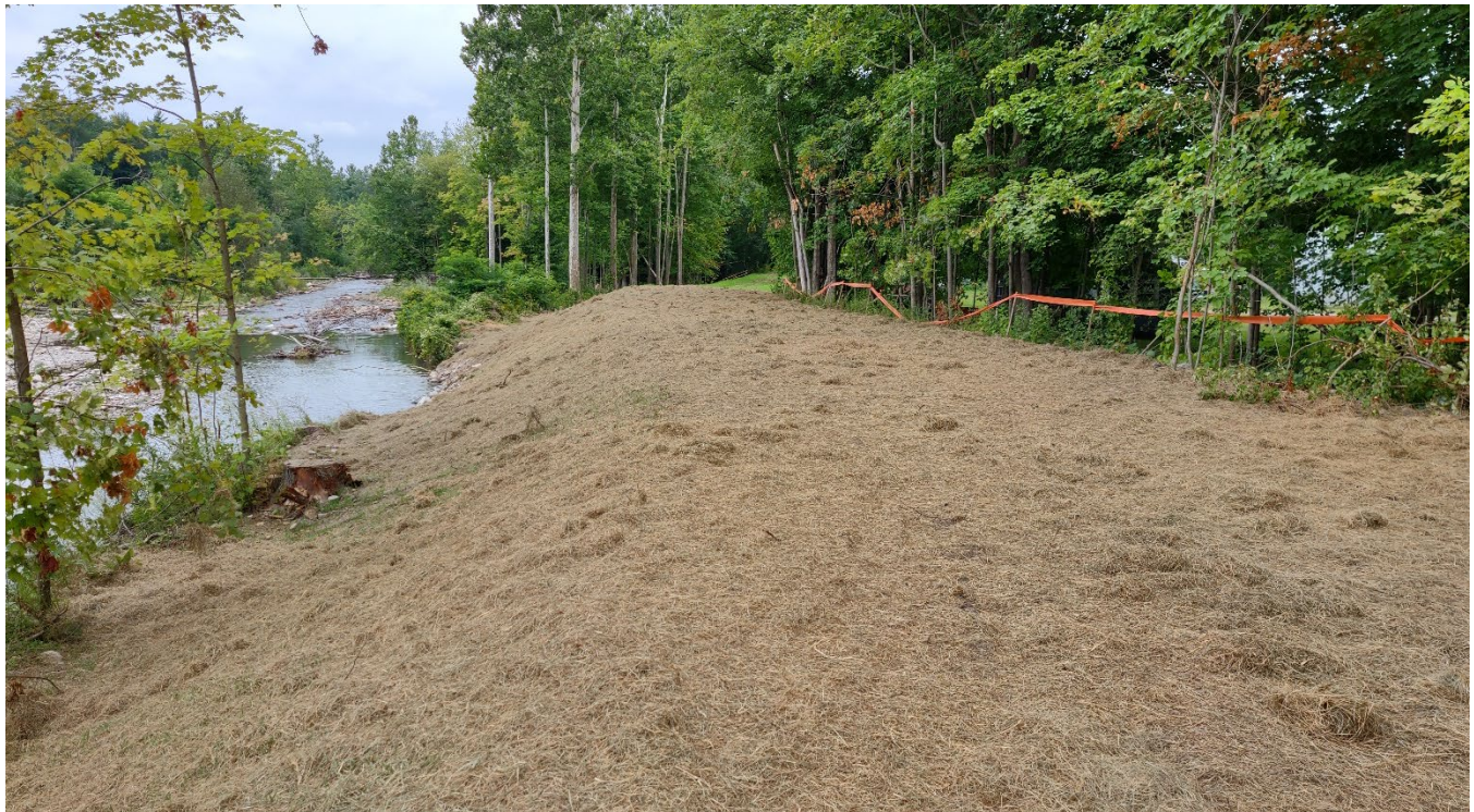
Figure 5: Work area at the Ossie Road Berm near the Murray parcel has been seeded and mulched.
