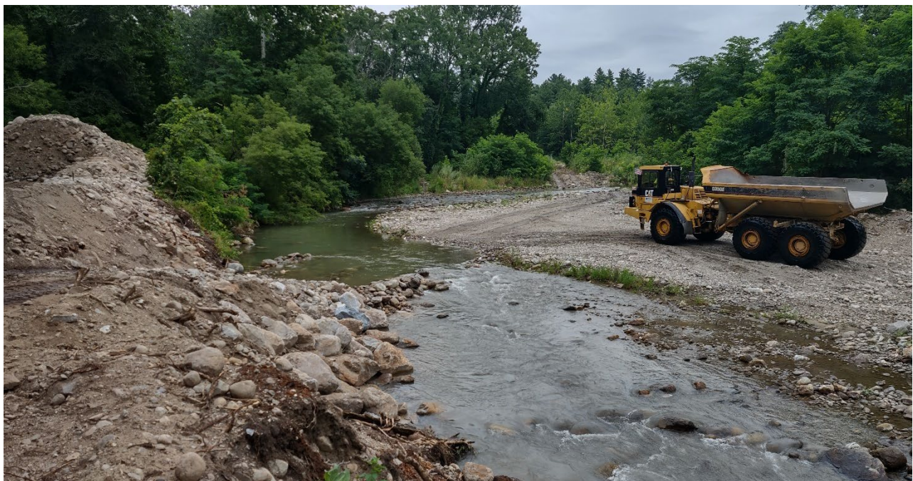
Figure 3: View of water crossing at the Goodro Lumber work site, two haul units transporting excavated sediment so that excavation work can be completed as soon as possible, and river crossings restored.
