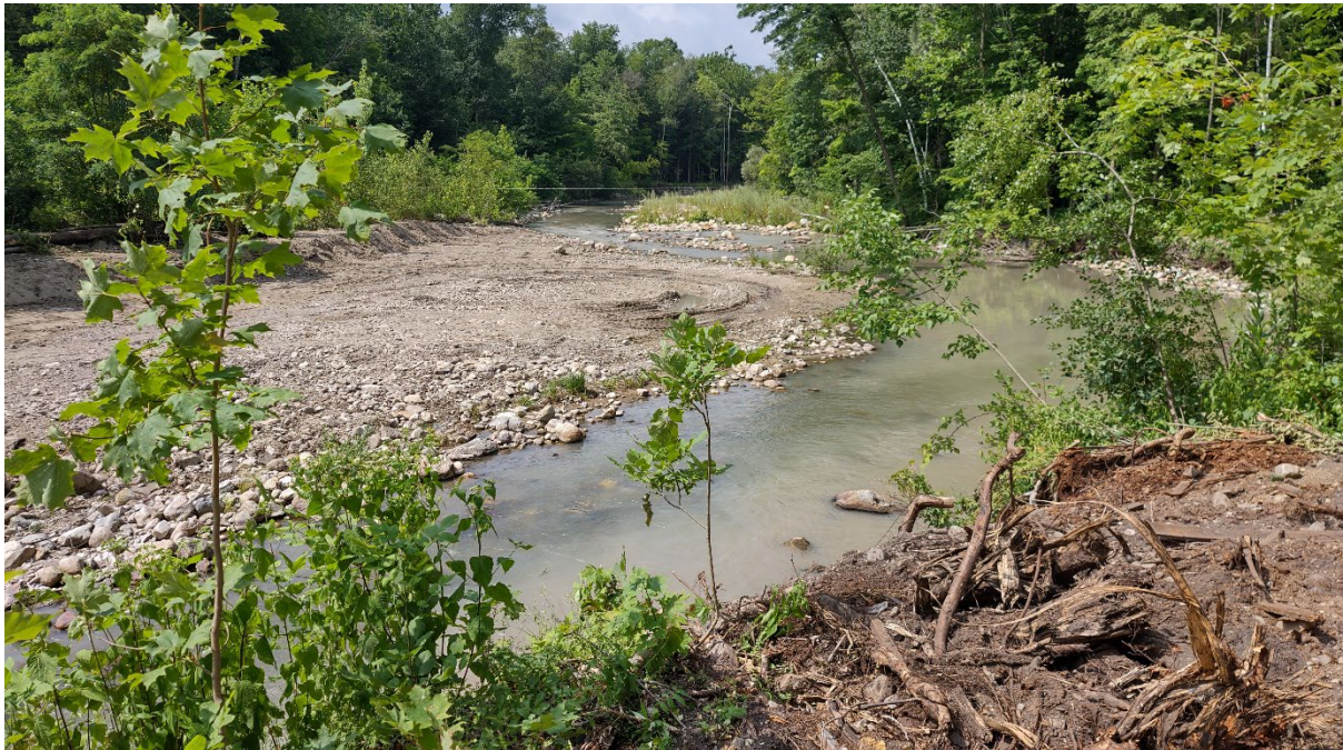
Figure 1: Sediment removal from Sediment Bar D, discharge of turbidity due to soft spot at water crossing visible in photo. Water crossing adjusted to avoid soft spot and minimize discharges.
