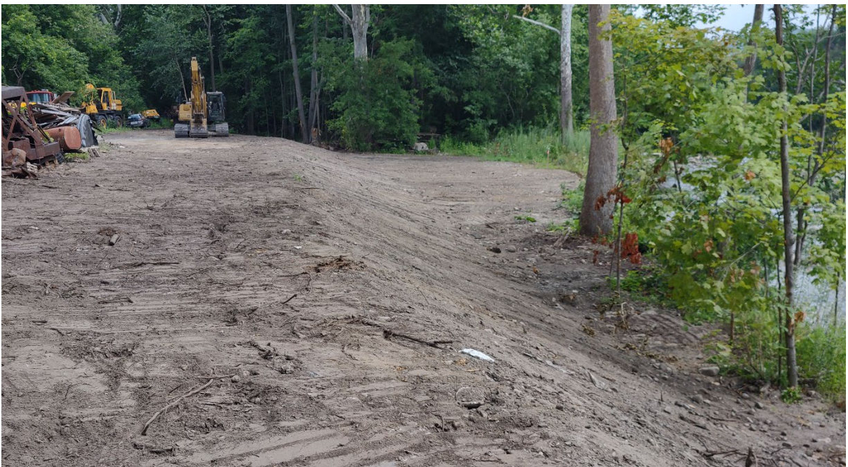
Figure 2: View of armored Ossie Road berm at the Murray parcel, topsoil and grubbings placed over the stone armoring, site awaiting mulch, live stakes to be planted at a later date.
