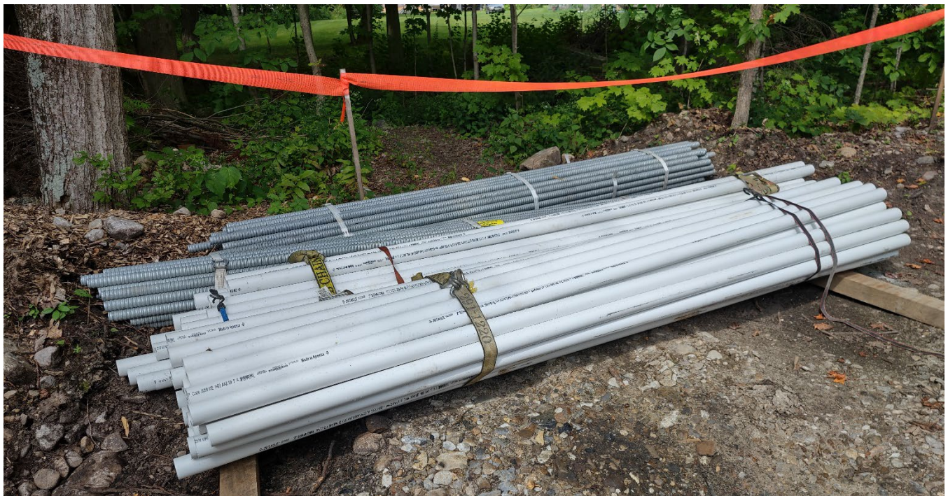
Figure 4: Ground anchor rods and PVC piping staged at the Grist Mill Road floodwall awaiting installation.
