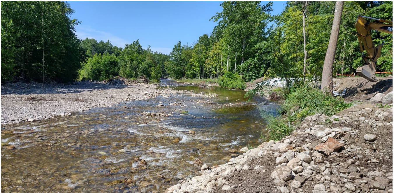
Figure 3: View of gravel bar after sediment removal looking downstream, flows remain higher than average for this time of year, with water flowing on the remaining edge of gravel bar.
