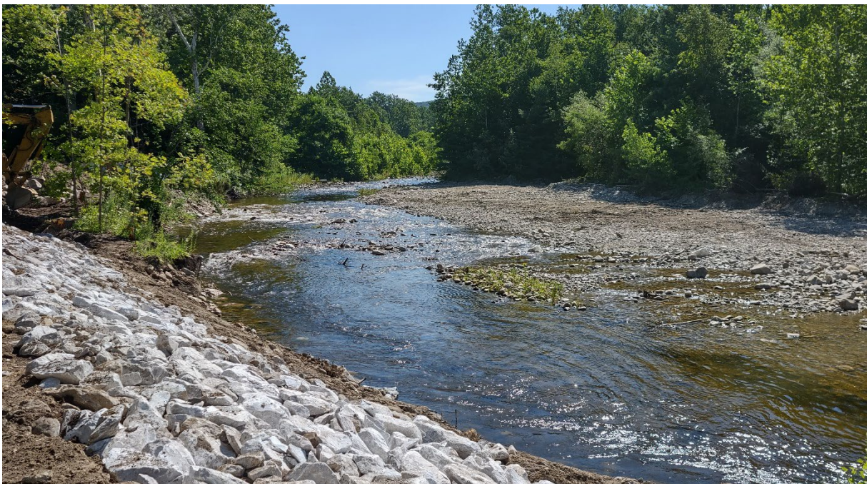
Figure 2: View of gravel bar after sediment removal looking upstream, flows remain higher than average, stone armoring in the foreground to be covered with grubblings, seed and mulch, and joint plantings.
