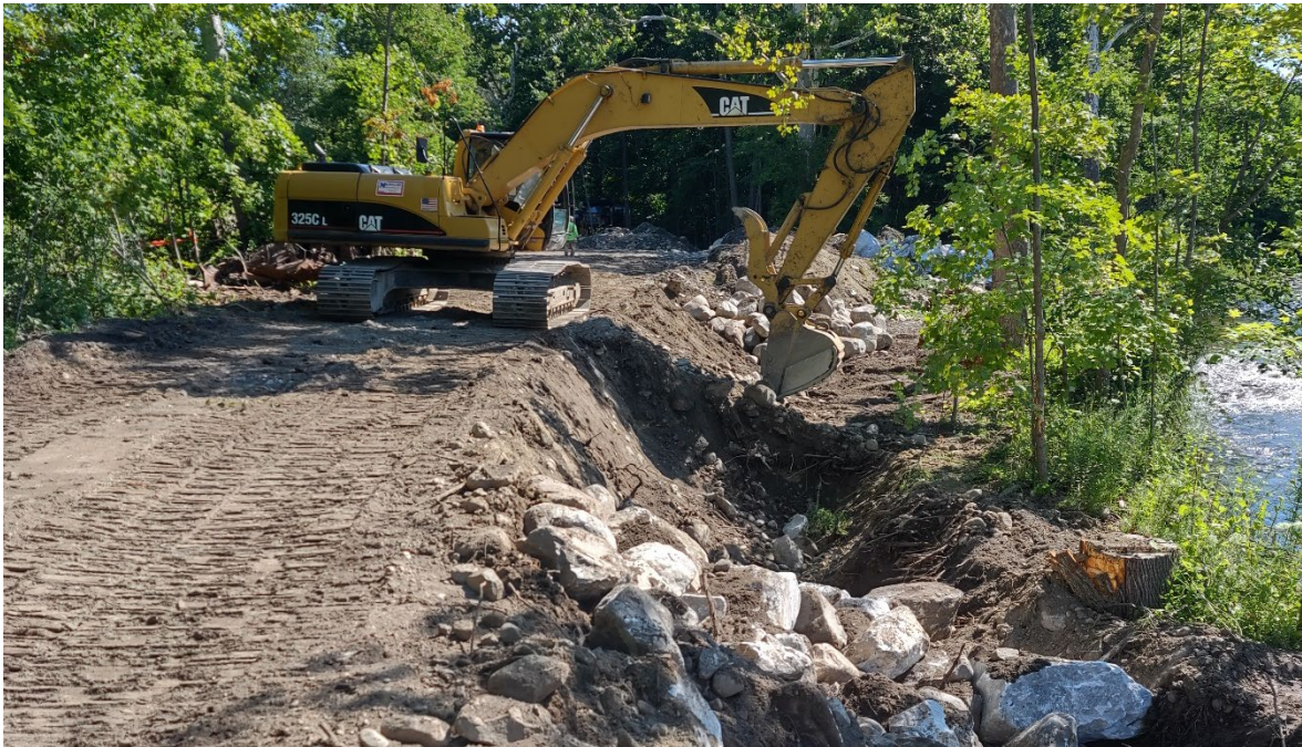
Figure 1: Stone armor installation at the Ossie Road Berm near the Murray Parcel.
