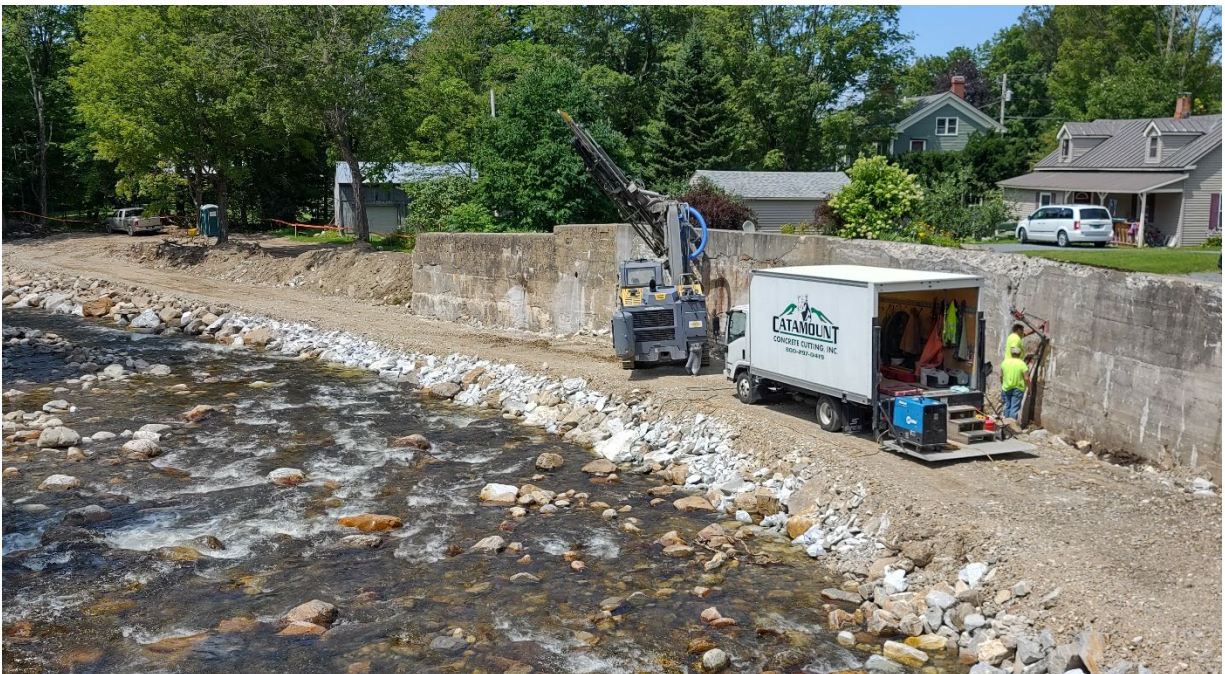
Figure 4: Concrete coring and rock drilling operation set up at the Grist Mill Road floodwall..
