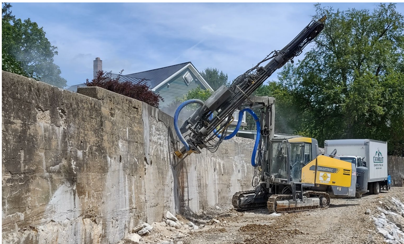
Figure 5: Rock driller completing holes at the Grist Mill Road floodwall.
