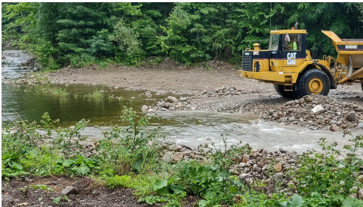
Figure 3: Flow has largely cleared within a minute after haul unit crossing.
