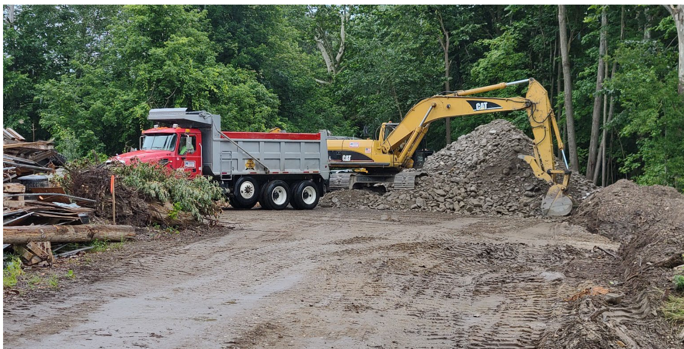
Figure 4: Excavated sediment being loaded into on-road dump trucks at the Murray parcel fill area.
