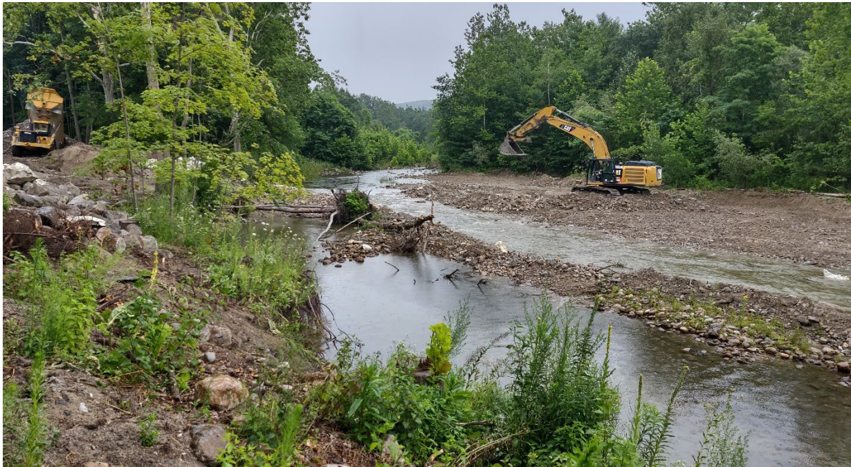
Figure 1: Sediment removal underway at gravel bar on the opposite side of river from Ossie Road berm, temporary isolation berm to keep flow from berm armoring work area visible in center of photo.
