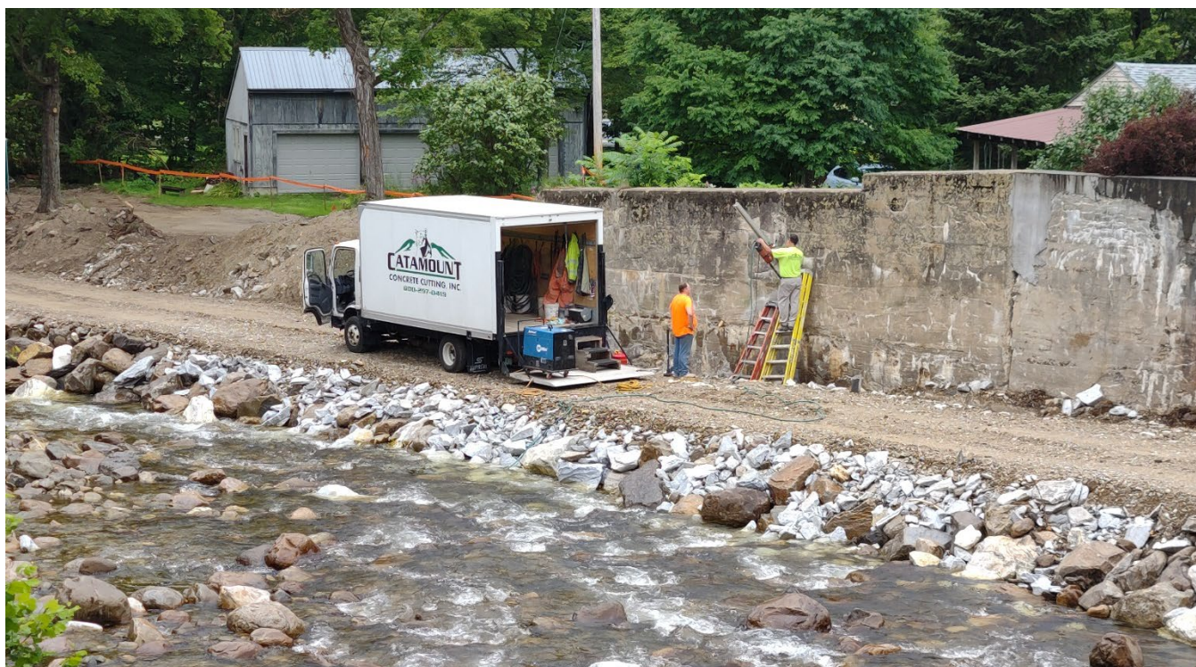
Figure 5: Coring operation underway at the Grist Mill Road floodwall.
