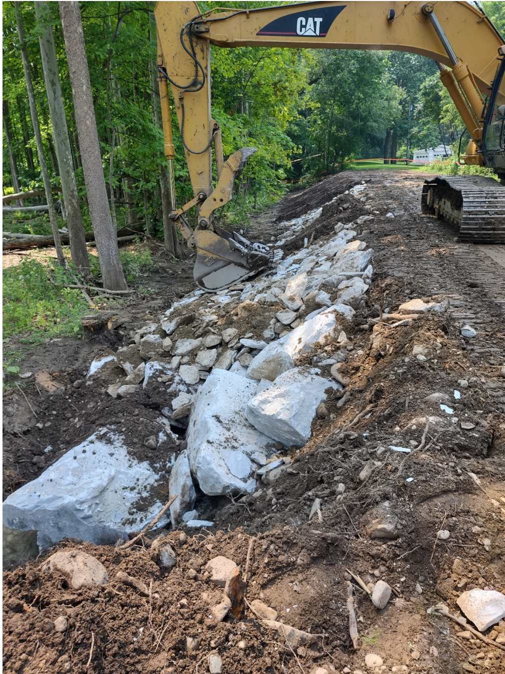
Figure 2: Installation of stone armoring along the Ossie Road Berm near the Murray parcel
