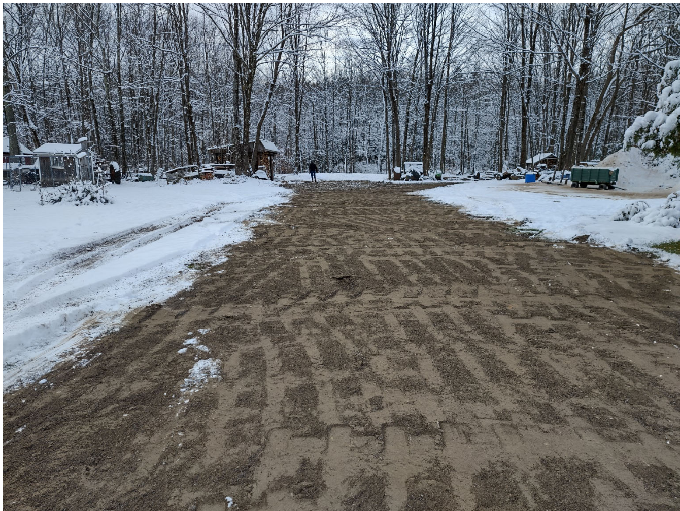
Figure 2: Installed topsoil following gravel access road removal at upstream site awaiting seed and mulch.
