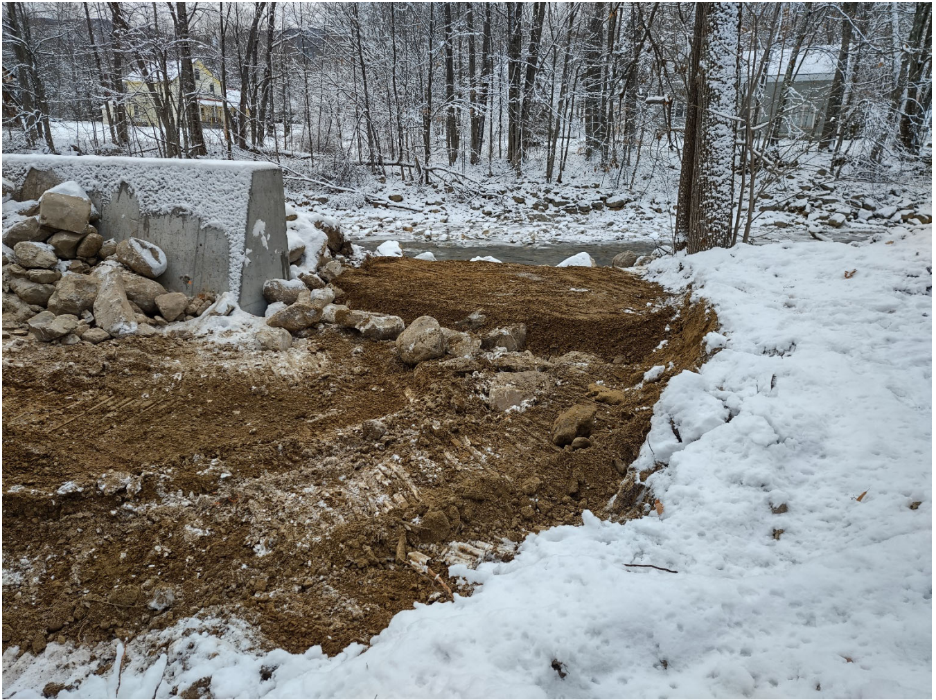
Figure 7: Placing stone fill and gravel at the flood wall opening to create elevated access and river viewing area. This approach allows future river access by the Town, while also meeting desires of landowners.
