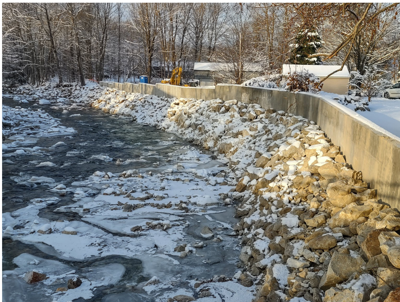
Figure 1: Final river setting with removed construction access road and replaced stone along flood wall.
