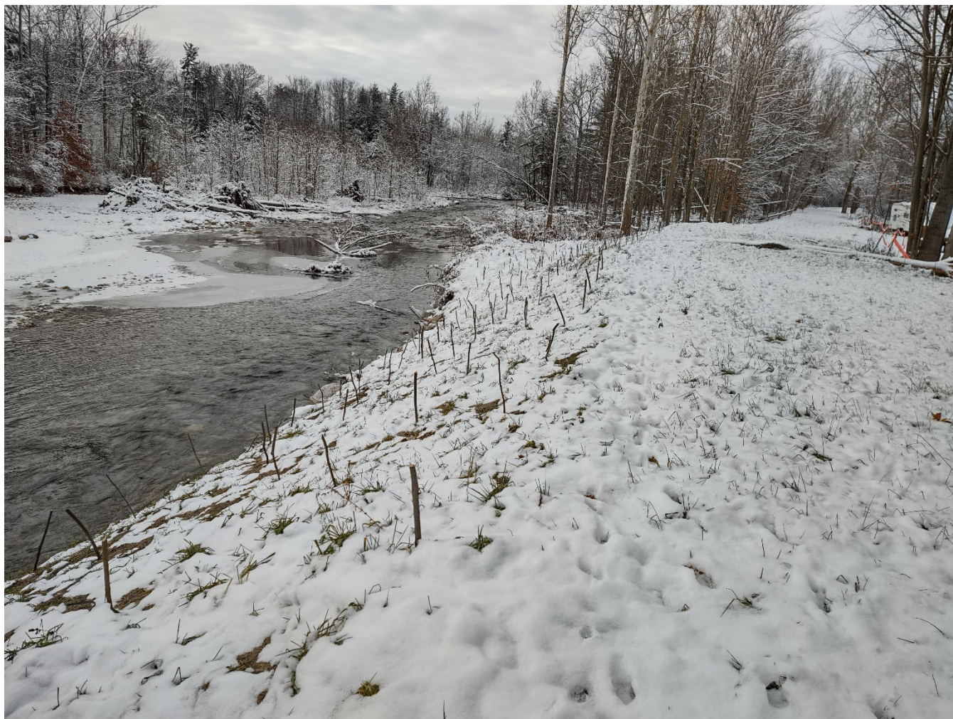
Figure 6: Installed dormant stakes at the Murray site.
