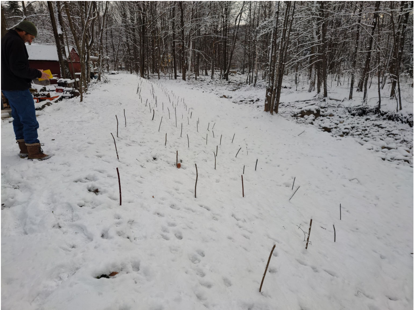
Figure 3: Installed dormant stake plantings at the upstream site along the armored slope. Note that these need to be driven in further.
