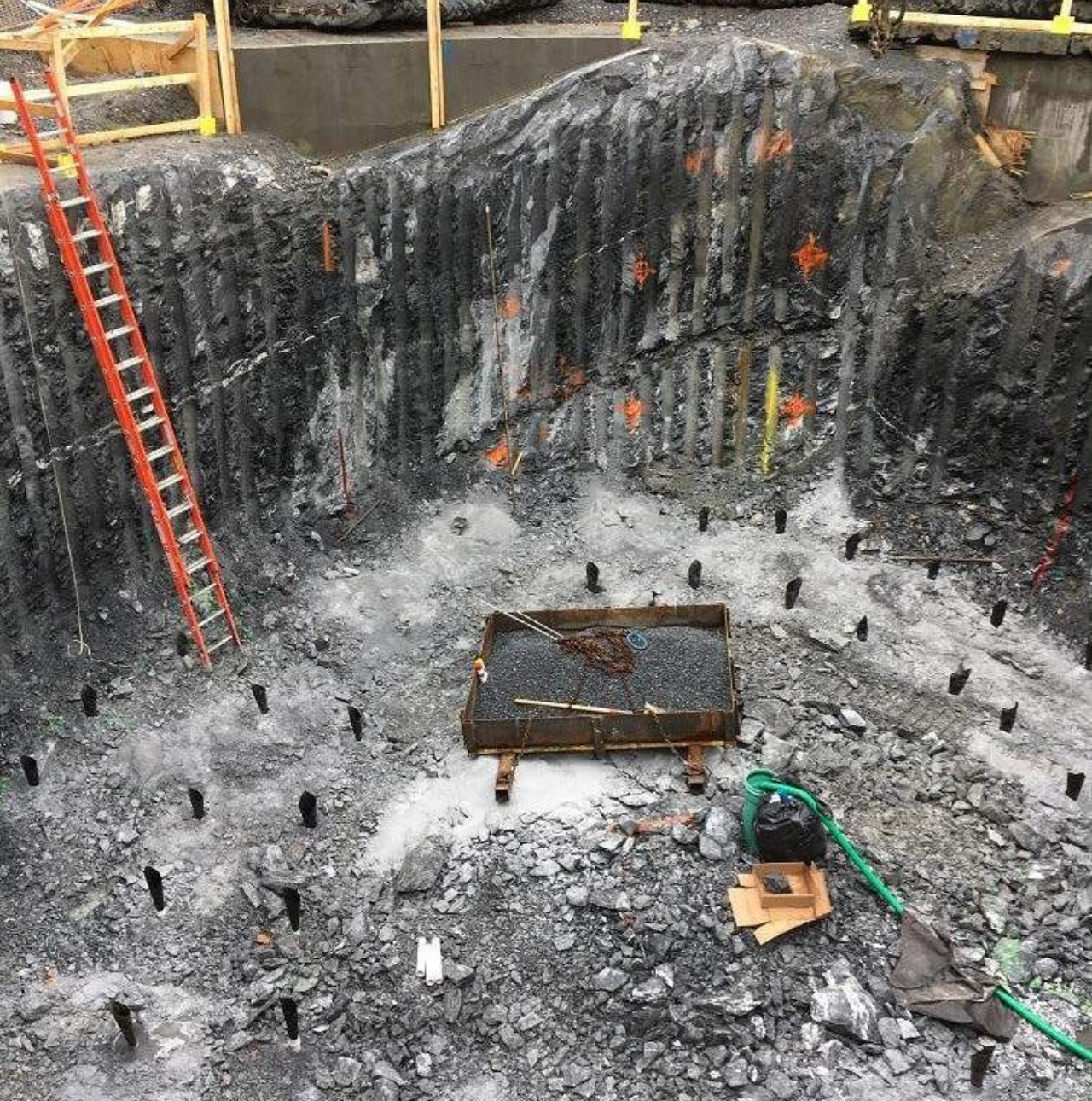
Microtunneling Launch Shaft Construction
