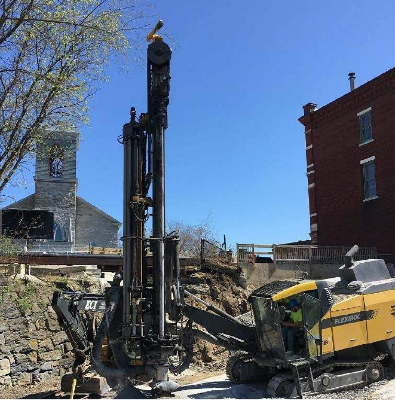
Microtunneling Launch Shaft Construction
