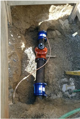
(Installation of new gate valve)
