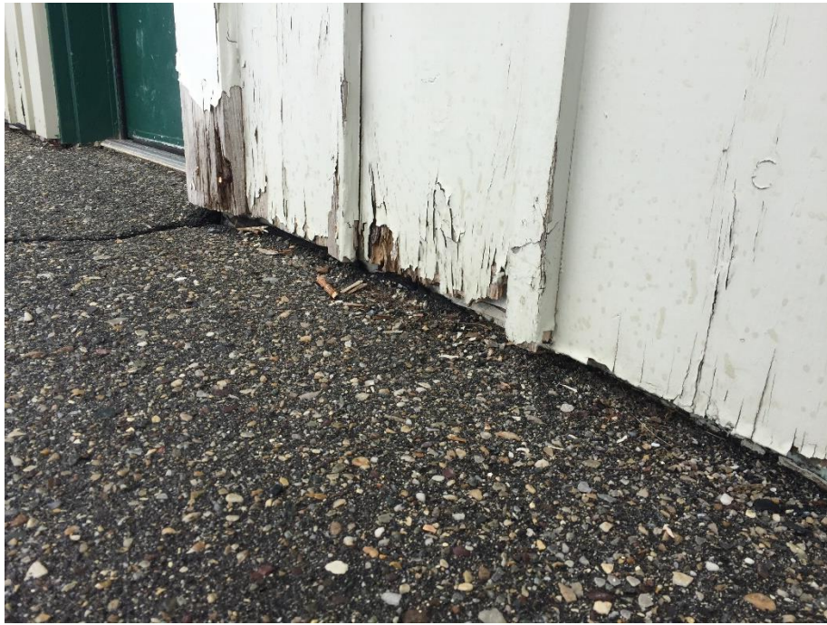
This is the section of the board and batten siding on the south elevation that has experienced rot damage due to how close it is to the pavement walkway.
