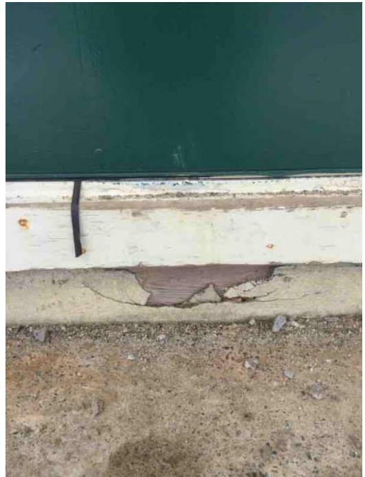
Damage to the stucco under the door on the east elevation.
