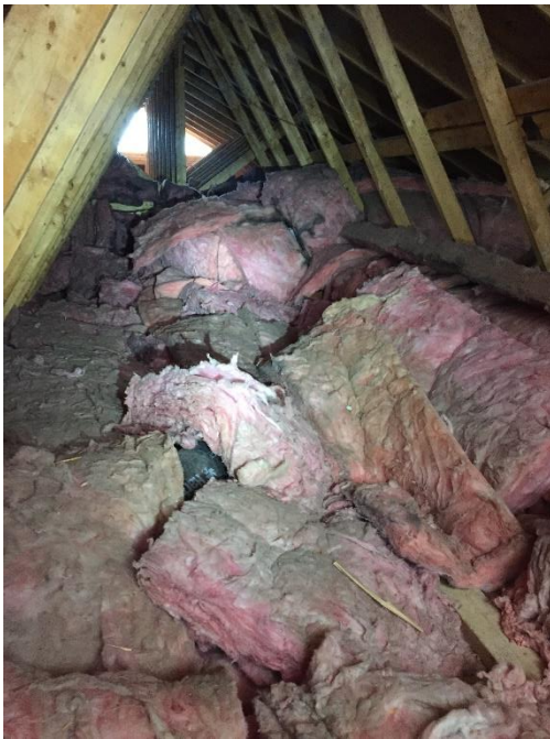
The current fiberglass batts insulating the attic are unevenly laid over top of joists and between the bays.
