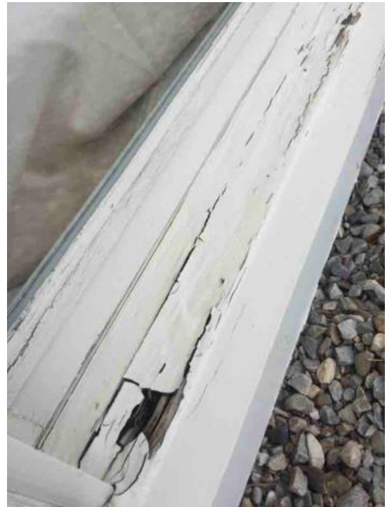
Seen here is a section of rotten wood and damaged EIFS at the north west corner of the building. Wood rot at the frame of a window sill.
