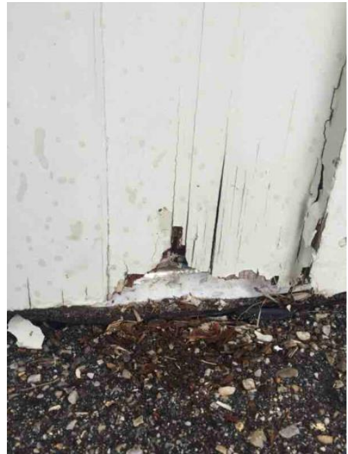
Moisture damage at the bottom of the siding on the south elevation over the pavement.
