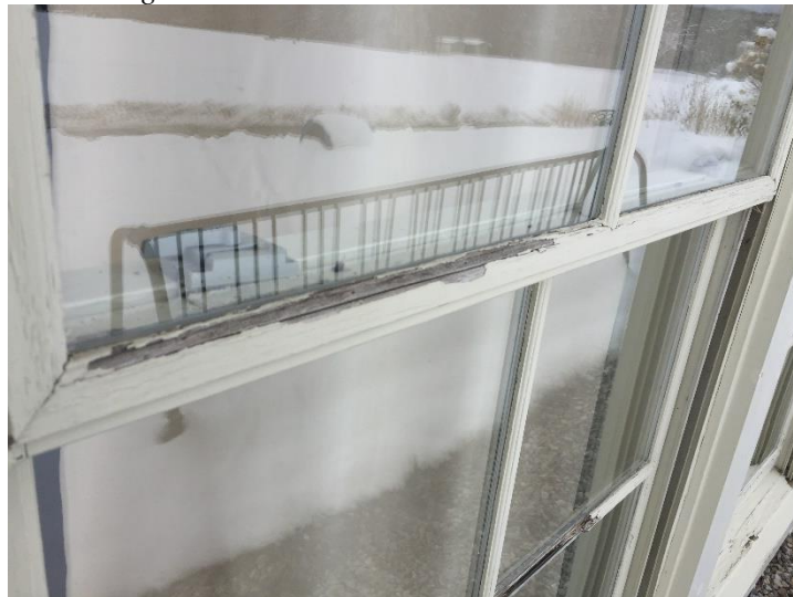
Horizontal surfaces which are not rotted are at risk for future rot where paint is peeling or missing.
