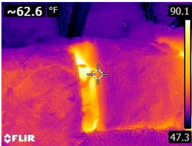
This image shows the heat loss from an uninsulated section of ductwork.
