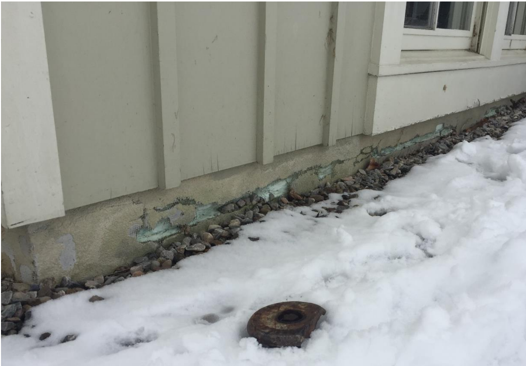
This image shows the damaged EIFS at the foundation on the north elevation. Seen here is exposed, damaged, and missing XPS (blue material.)
