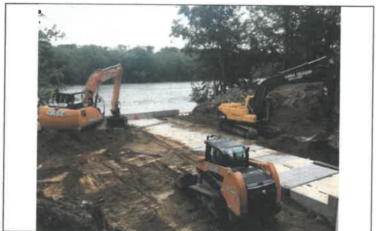
South River Street Precast Concrete Culvert
