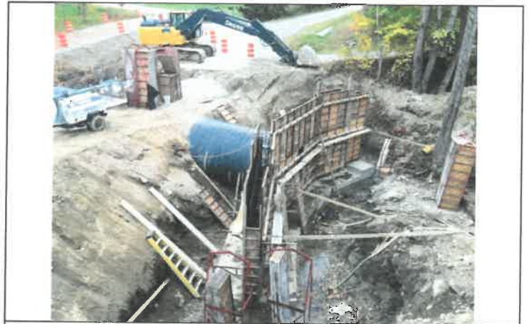
Collins Mountain Road Outlet Headwall
