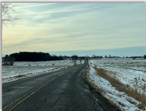
Figure 1: Eastern end of Cady Road looking east
