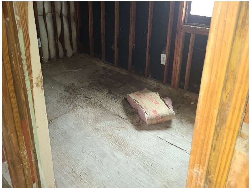
Photo 2: Water damaged and broken plywood
