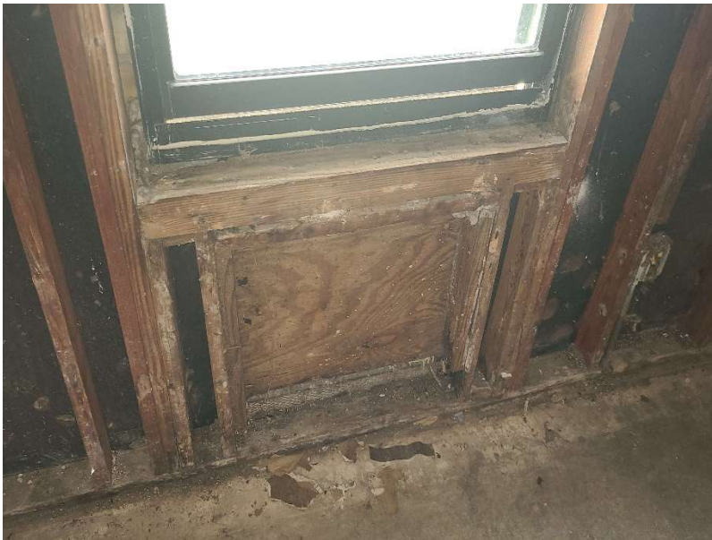
Photo 8: Rotten framing around window
