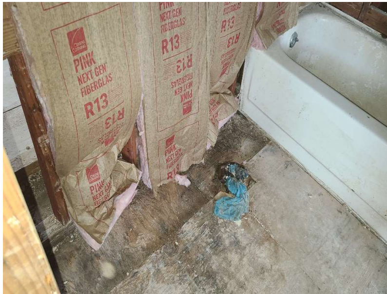
Photo 5: Rotten plywood and framing members in upstairs bathroom
