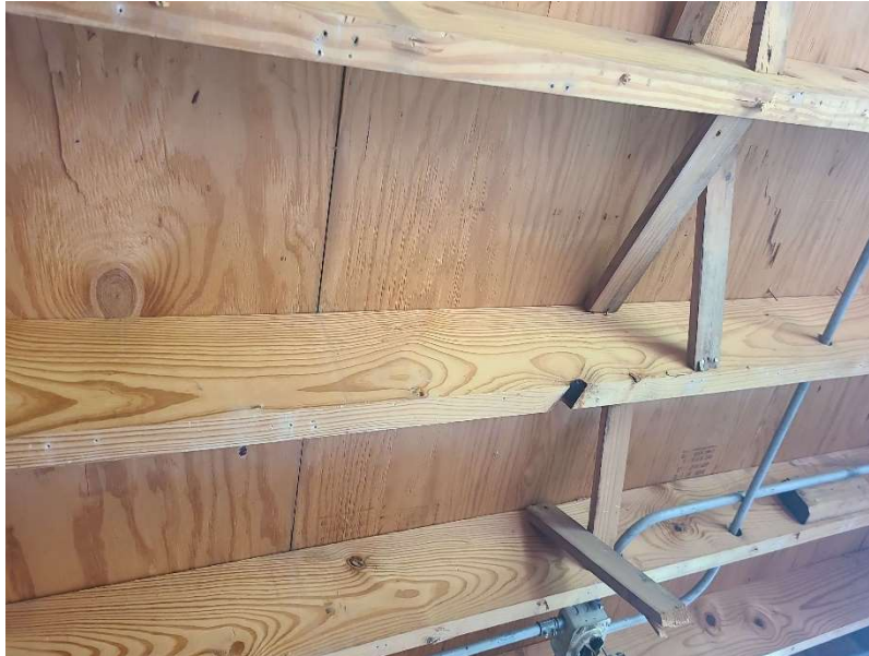
Photo 1: Broken plywood and blocking not attached
