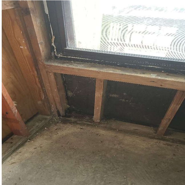
Photo 13: Rotten framing under window
