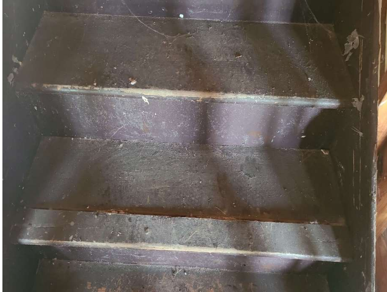
Photo 3: Broken stair tread
