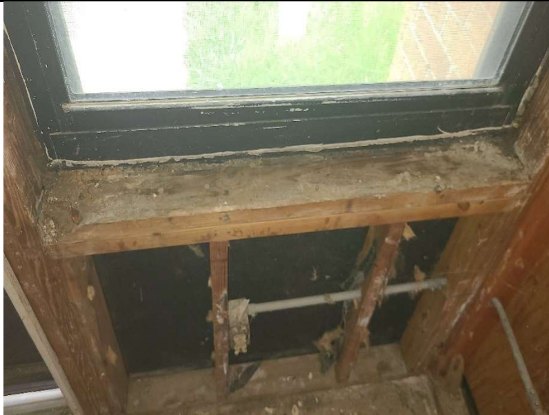
Photo 7: Rotten framing around window
