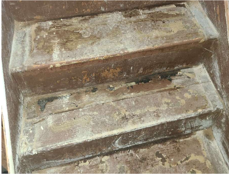
Photo 1: Broken stair tread
