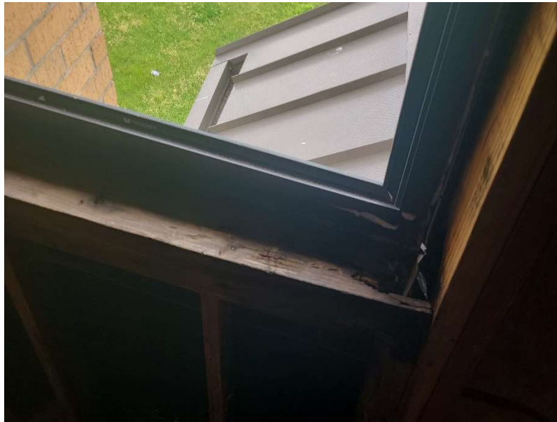
Photo 5: Rotten framing under window
