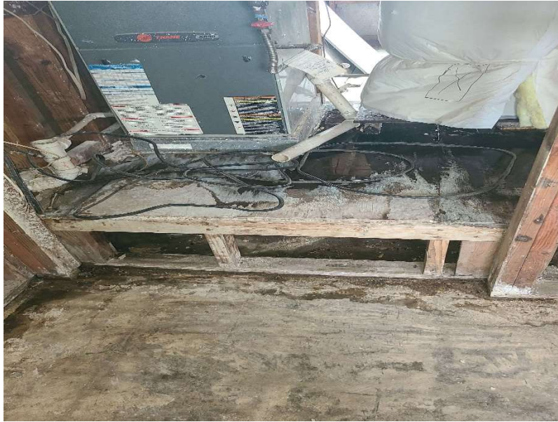
Photo 5: Leaking water heater, plywood and framing rotten
