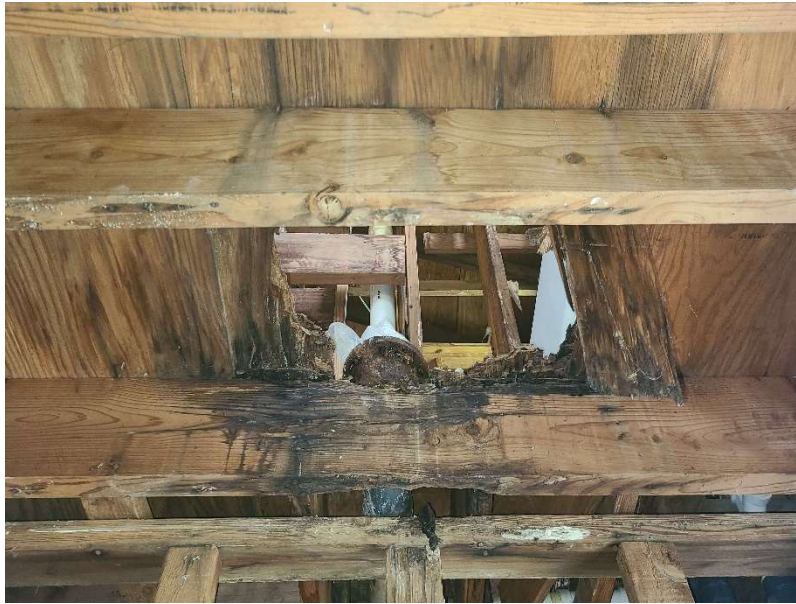
Photo 3: Rotten plywood and framing above kitchen
