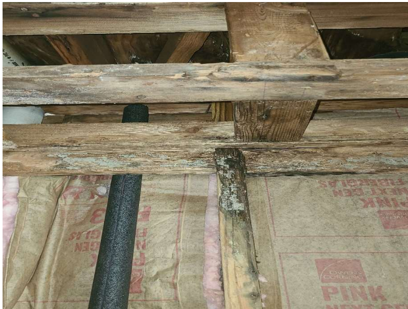
Photo 4: Rotten framing above in kitchen
