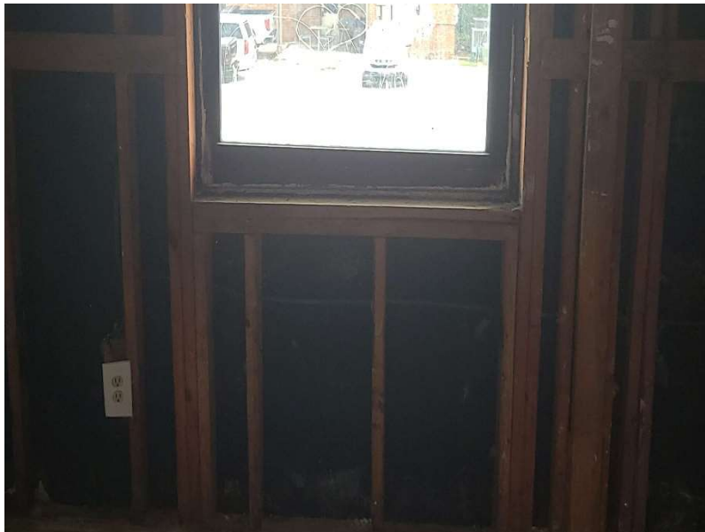
Photo 4: Rotten framing around window
