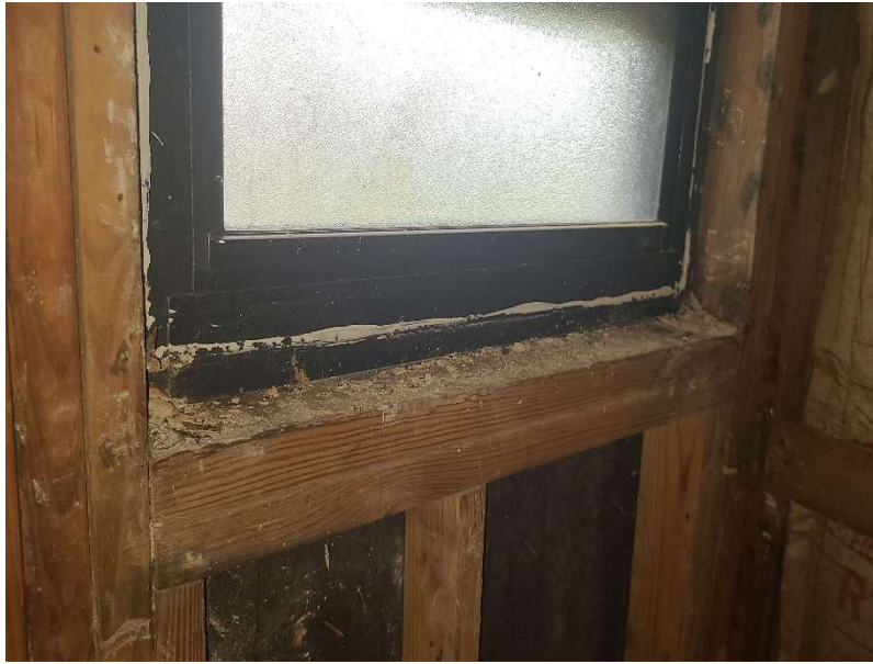
Photo 15: Framing at window rotten
