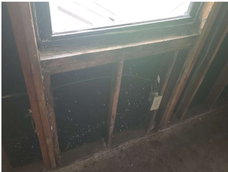
Photo 6: Rotten framing around window
