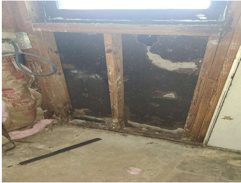
Photo 11: Rotten framing under window
