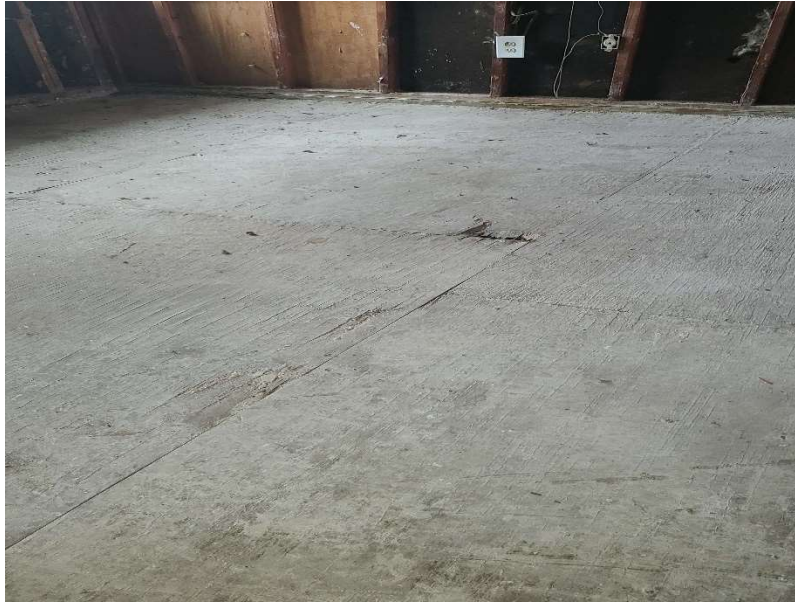
Photo 3: Broken plywood, typical throughout entire second floor
