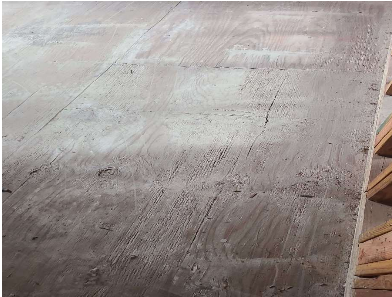
Photo 7: Broken and unsalvageable plywood on second floor
