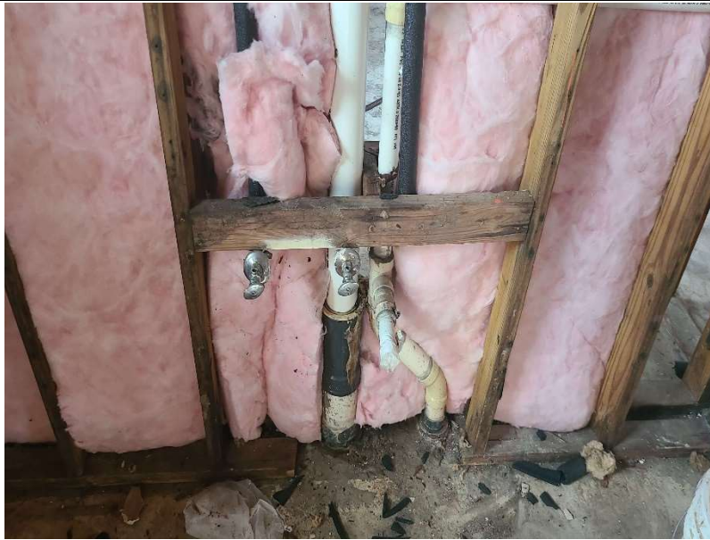
Photo 1: Rotten wood below in kitchen
