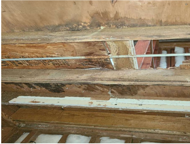
Photo 9: Water damage on plywood and framing members from below
