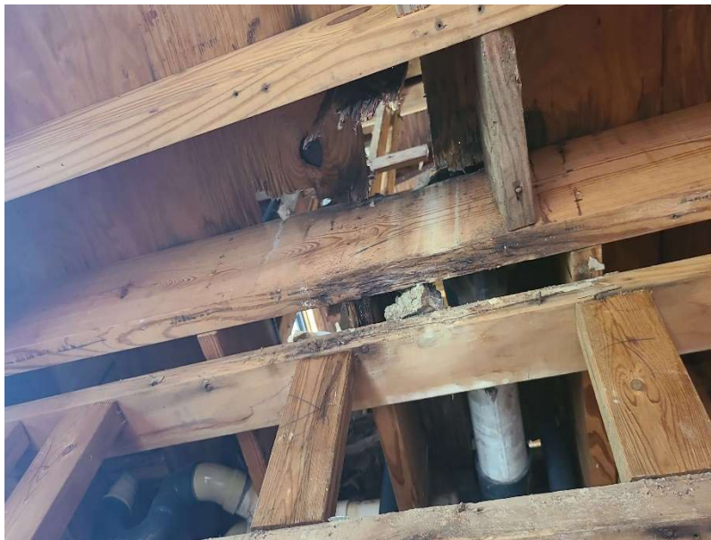
Photo 2: Rotten plywood and framing above in kitchen
