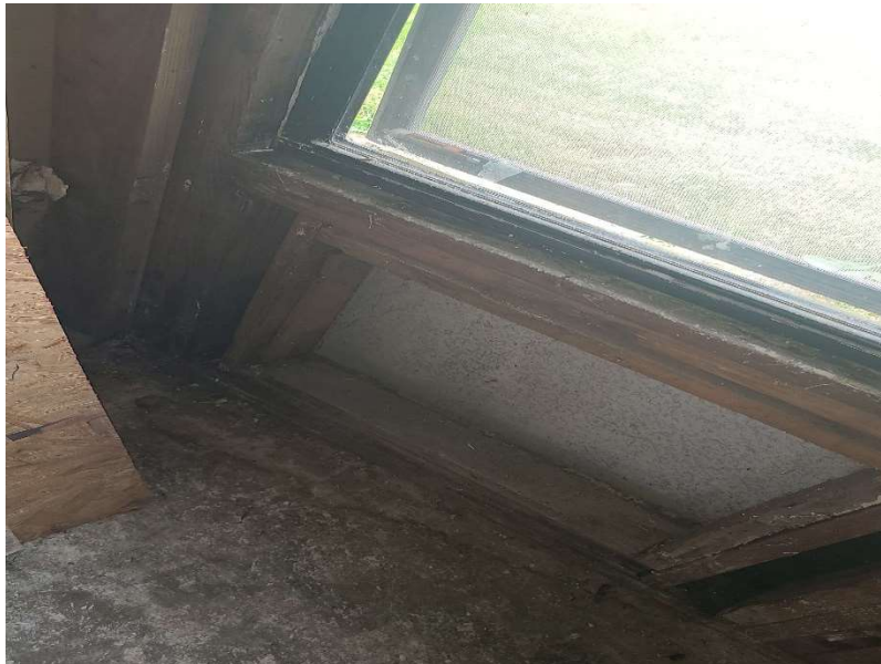
Photo 2: Rotten framing around windows
