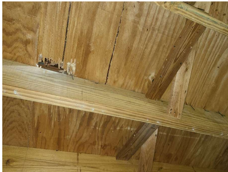
Photo 6: Broken plywood on second floor from below
