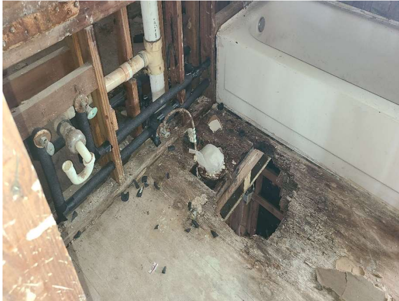
Photo 7: Framing members and plywood rotten in upstairs bathrrom
