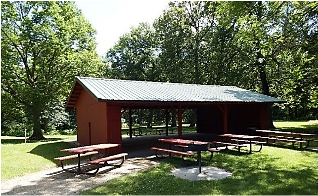
Stahl's Lake County Park picnic shelter with gravel pathway visible.
