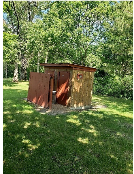
Swan Lake County Park restroom facility.
