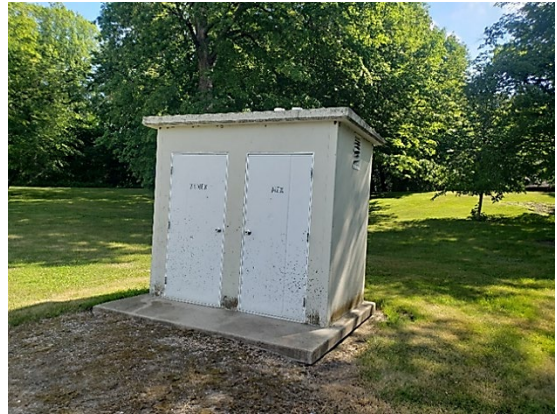
William May County Park restroom facility.
