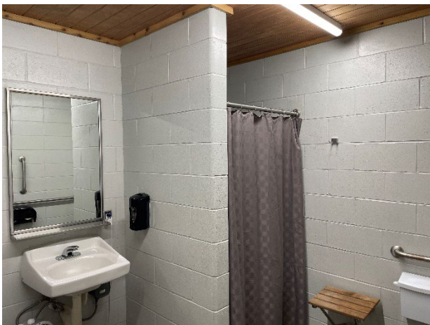
Interior of Piepenburg Regional Park campground shower facility.
