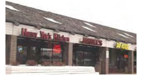
Figure 13. Skylights are discouraged in applications such as in the photo.
