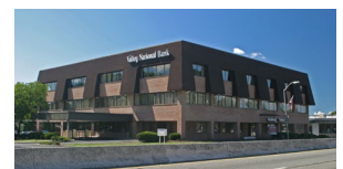
Figure 12. Mansard roof designs are prohibited.
