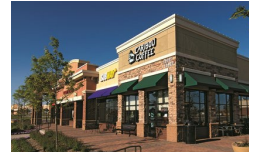
Figure 3. Good use of pilasters, varying rooflines, building materials, awnings and projections.
