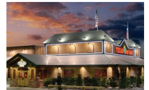
Figure 6. Faux roof structures should be used to break up the mass of the building and to screen roof-top mechanical units.
