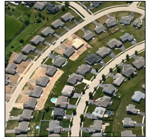
Figure 6: New residential construction in the northeast portion of the Village.
