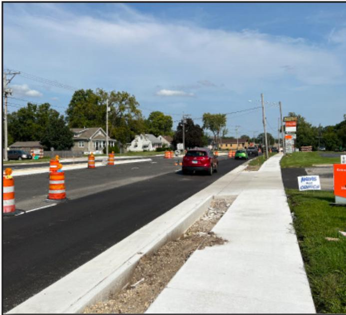
In addition to our Harlem Road project, the Village also reconstructed Indigo Lane, adding a new pavement surface, curb and gutter, storm sewer, and sidewalks along the west side of the road. This project was completed ahead of schedule and the final course of asphalt will be placed next summer, which will allow for settling to take place during the winter months. Darwin Drive, between Norman Avenue and China Berry Lane, is also being constructed this year.
