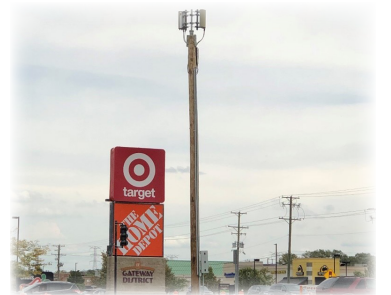
Small Cell Wireless Facility on the NW corner of Alpine Rd & Rt 173
