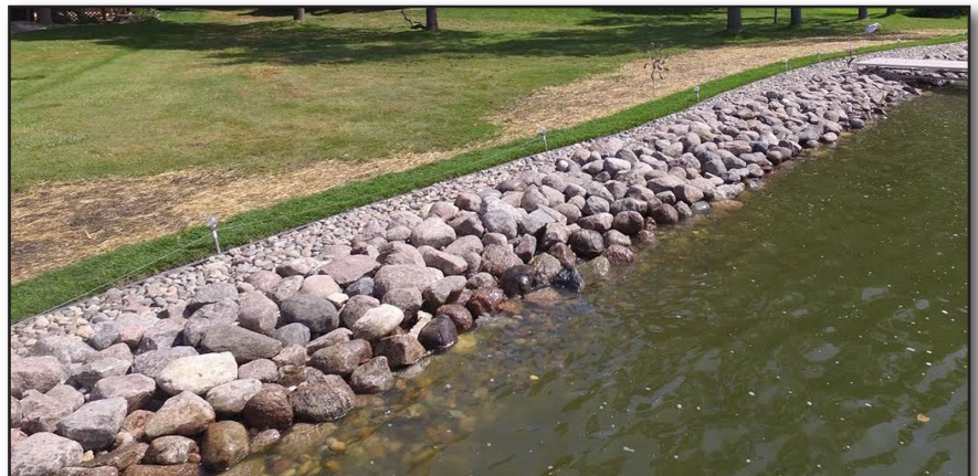
Example of acceptable Bank Stabilization using rip rap.
