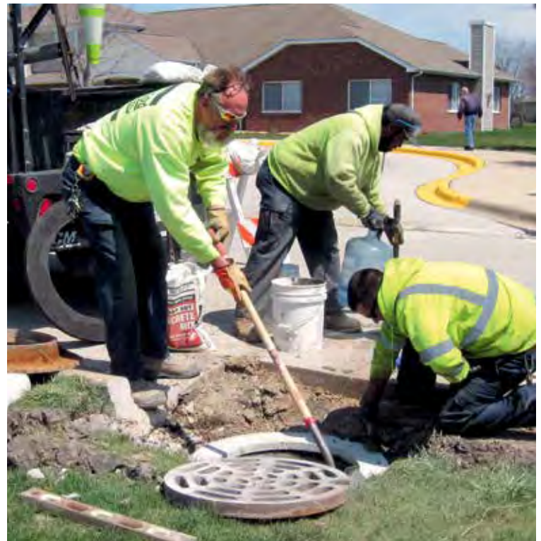
One of the Public Works Department's seasonal projects is sewer curb drain repair. Working on a curb drain are (left to right) crew leader Rob Boehl and Department employees Sylvester Robinzine and Dan Lebeter. The project continues through the warm weather months.
